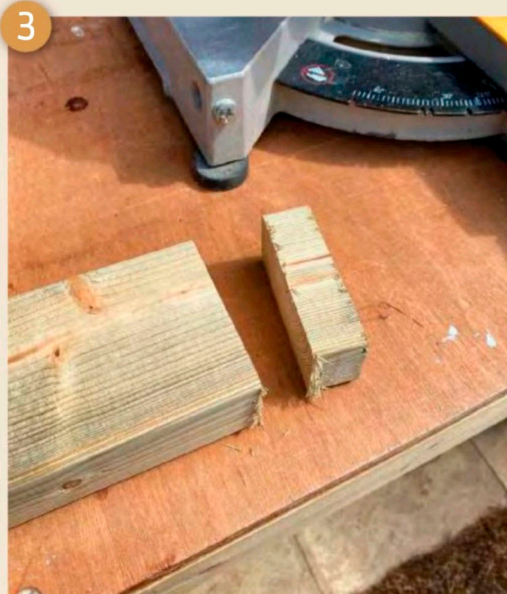
Before cutting anything to size, take the ends off each piece of timber
