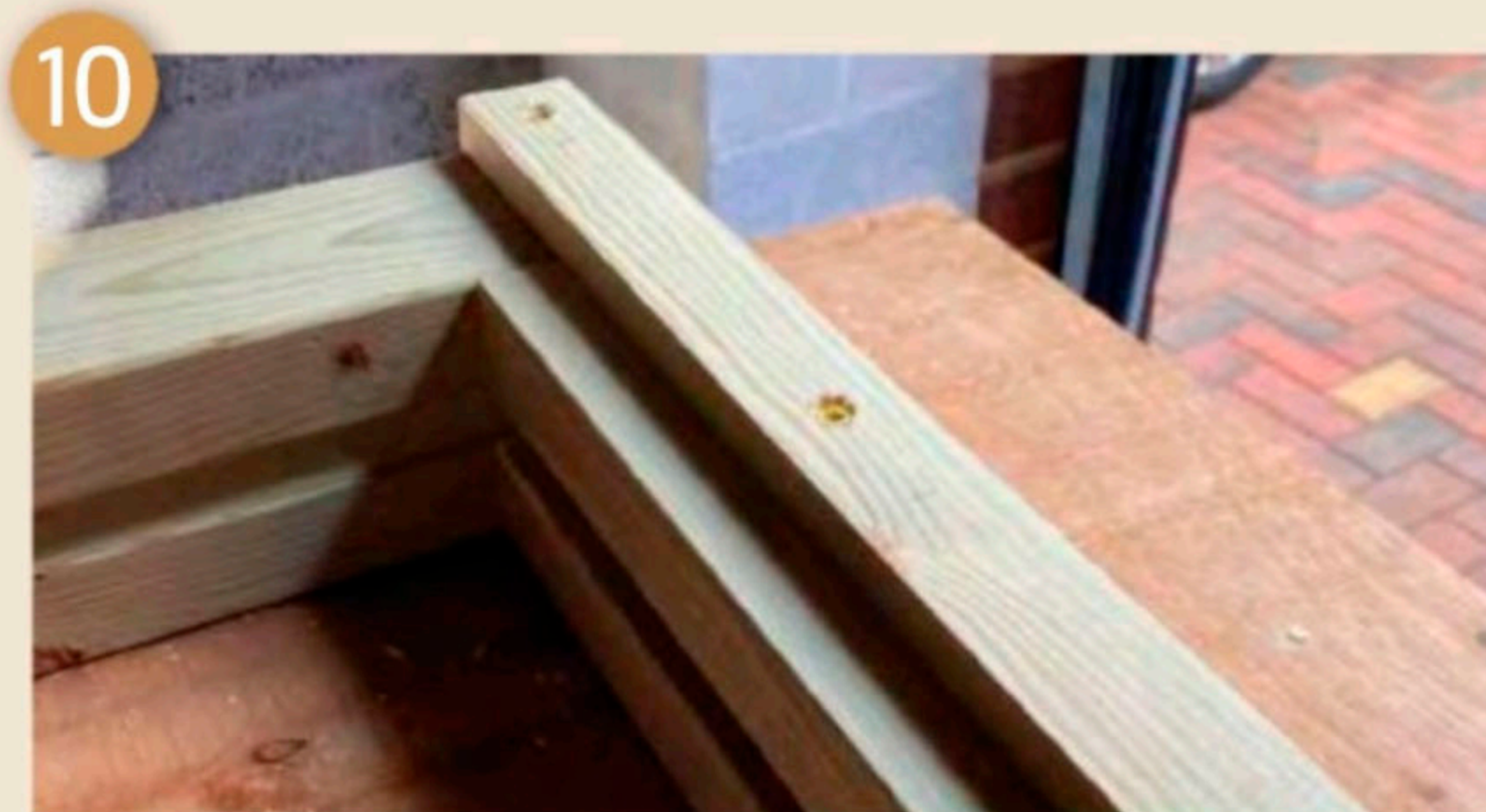
Join these together with three wood screws
