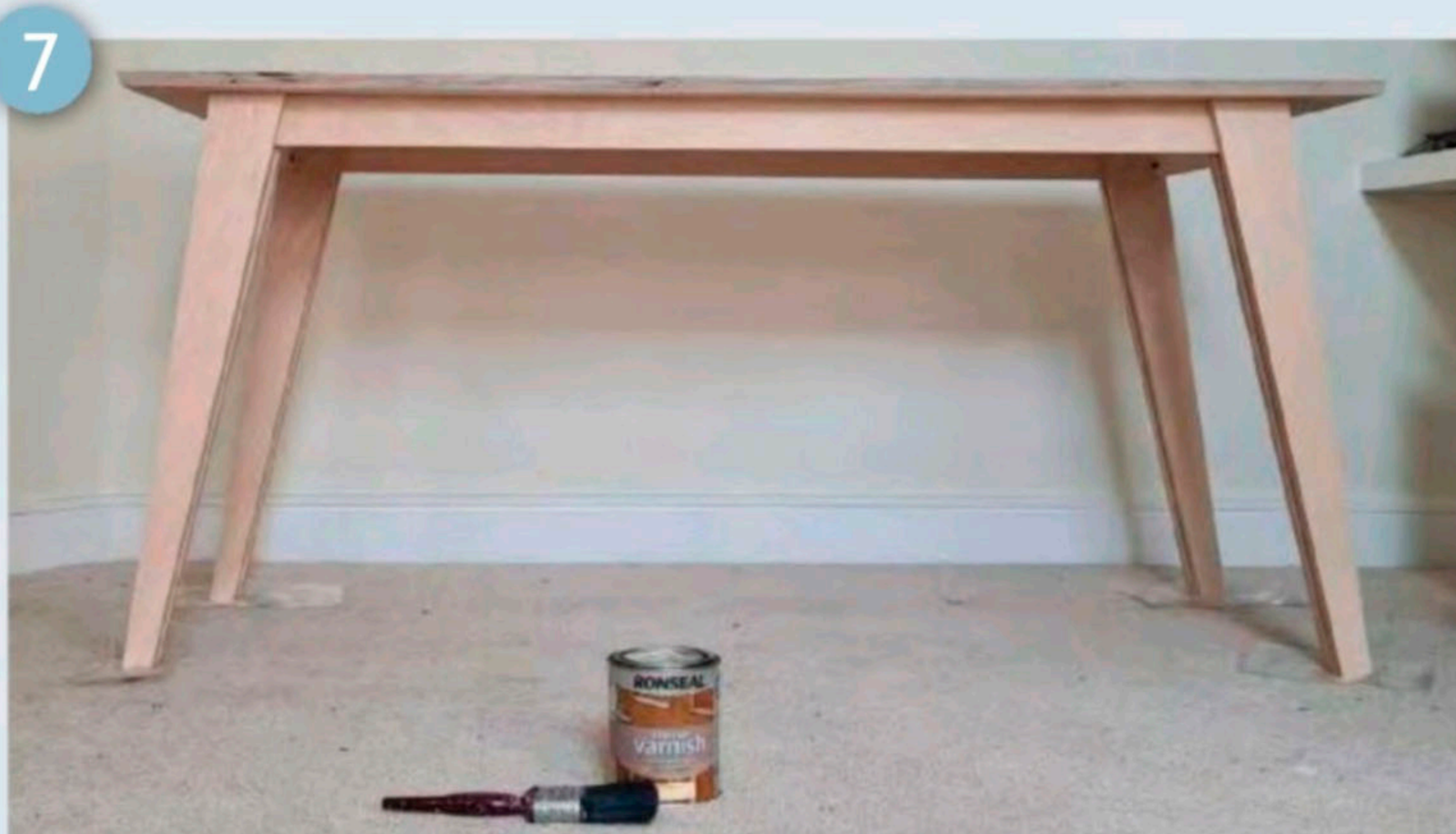
Apply polyurethane for a smooth finish
