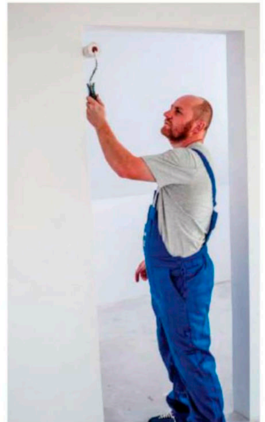
Before the pros paint walls, they fill holes and patch cracks with joint compound
