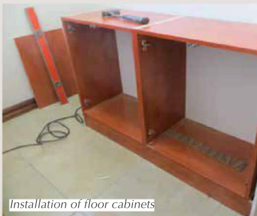
Installation of cabinet
