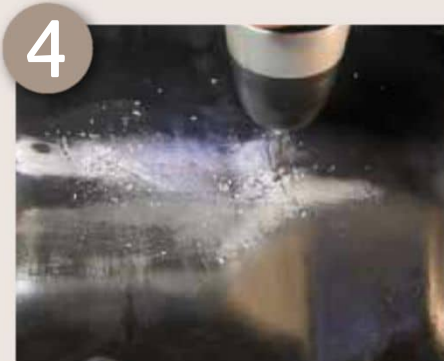
Drill two small holes on either side of the crack
