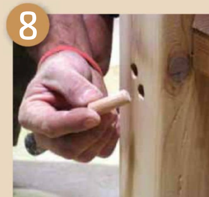
8 Fill in nail and screw holes with dowels
