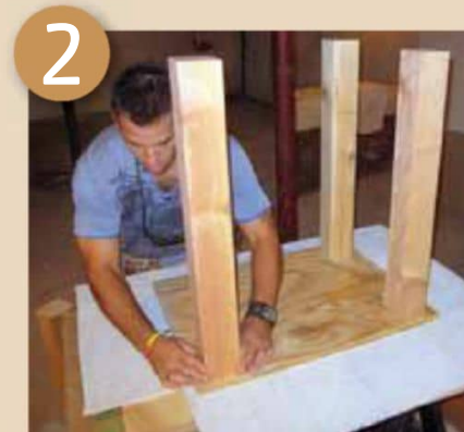
2 Position the legs on the plywood
