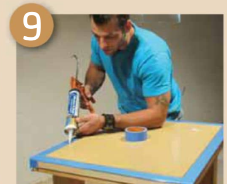
9 Run a silicone bead between the wood and cutting surface
