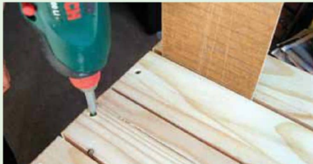
Fig. 15: Fitting the base slats
