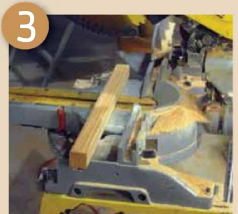
Cut supports for the leg
