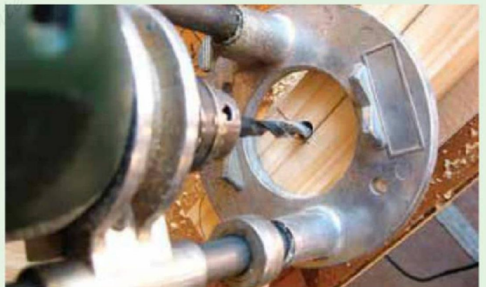
Fig. 4: Drilling the jigsaw pilot holes
