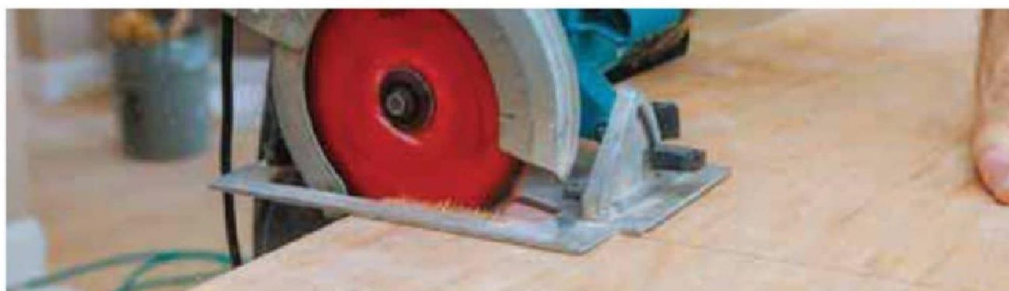
Cutting plywood with a circular saw
