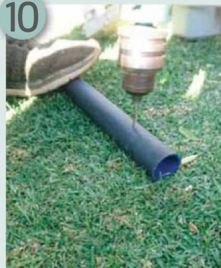
Drill holes in the steel bars
