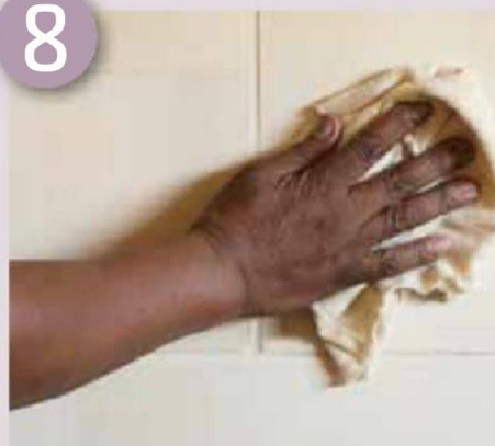
Polish the tiles with a clean cloth
