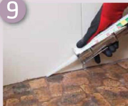
Seal the perimeter joints of the shower with a silicon sealer
