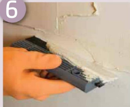
Apply the grout
