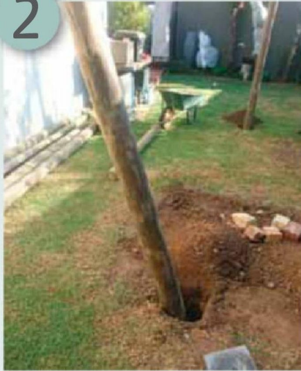
Holes dug and uprights in
