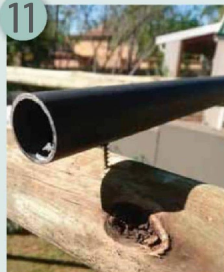
Fit steel bars to the beams
