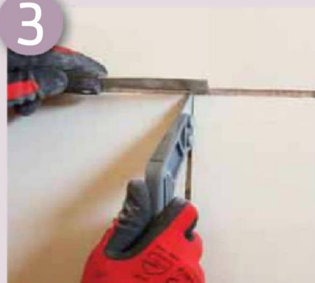
Remove existing grout
