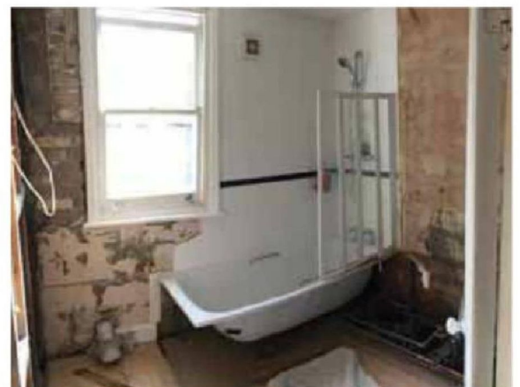
This is how this bathroom looked like partly demolished. There was a lot of existing pipework running above the floor that needed to be altered. Walls and floor were out of line and level and not suitable for good quality finish. Existing floorboards were also not suitable for tiling.
