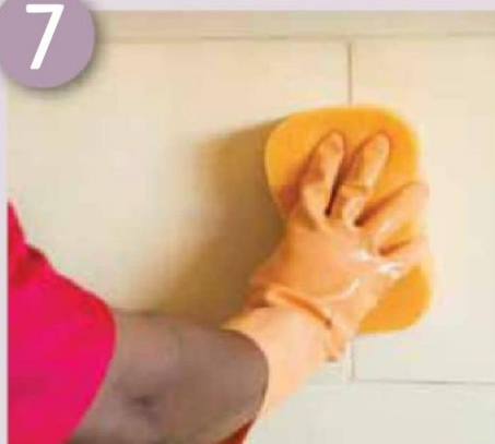
Clean off any excess
