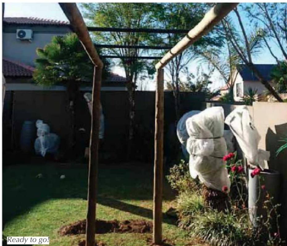
Fit steel bars to the beams
