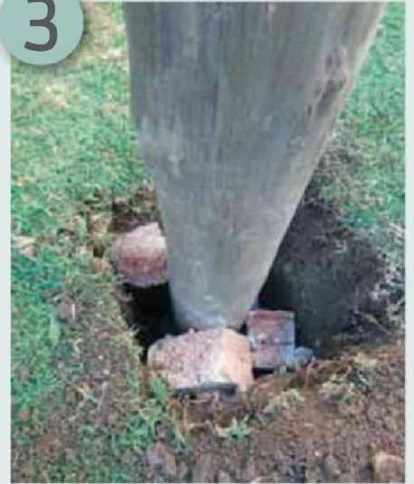
Support the uprights in the holes
