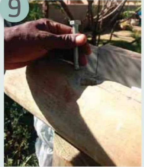
Securing the beams to the uprights
