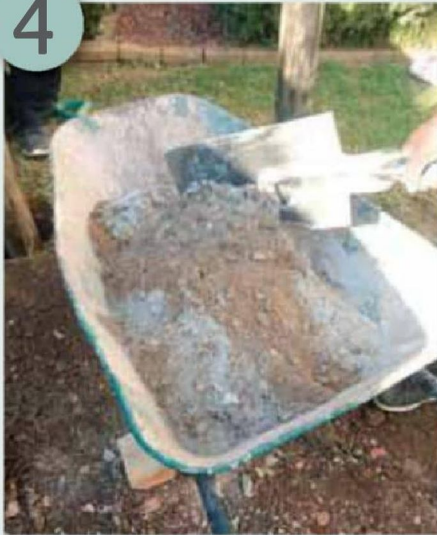
Mix your concrete
