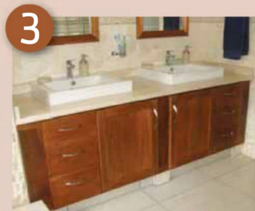
Finished vanity unit
