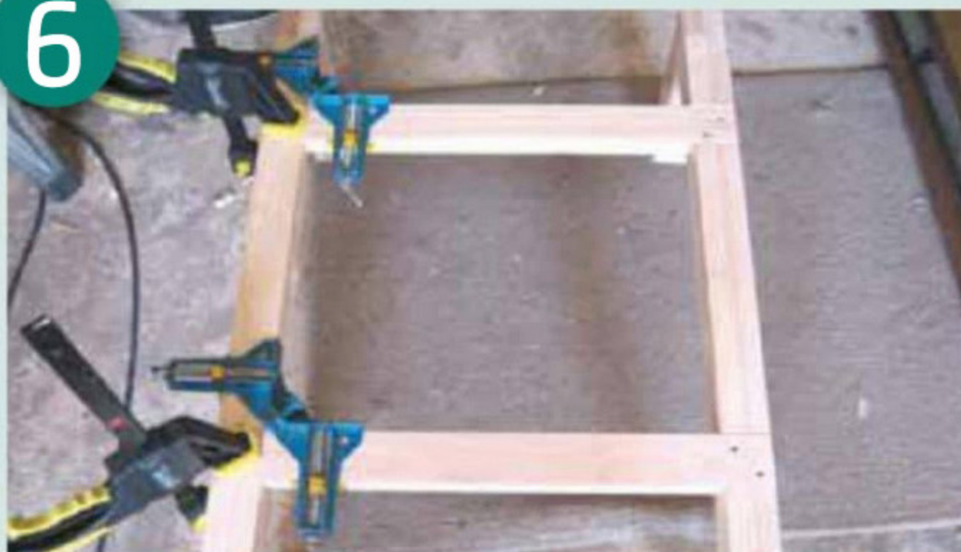
Clamping the cross supports
