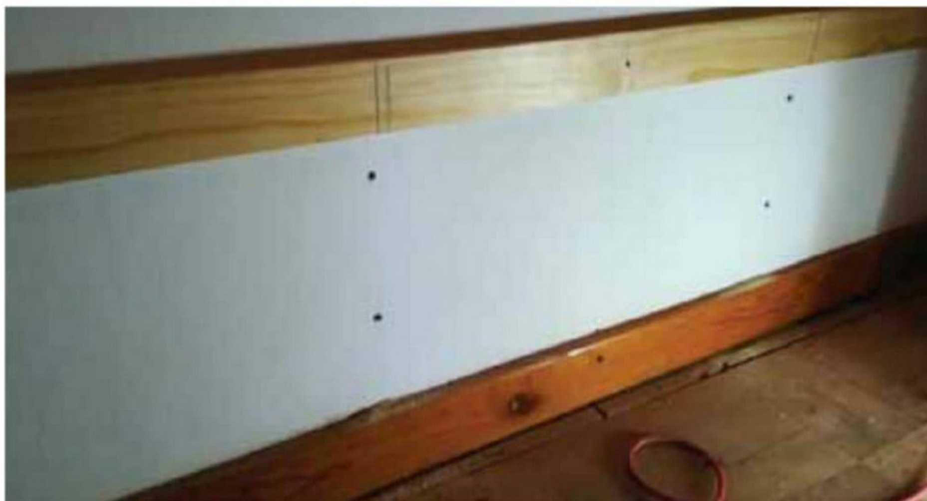
Story stick in place for lowest shelf. The holes below the stick are as drilled through the bracket, those above have been opened for the wall plugs
