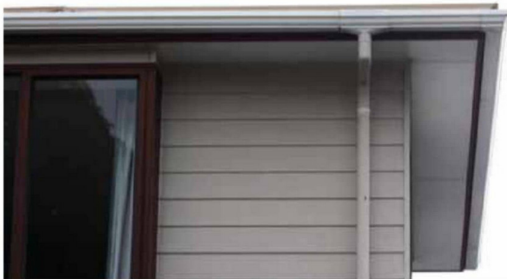
Gutters and downpipes require regular cleaning, especially if leaves fall into them
