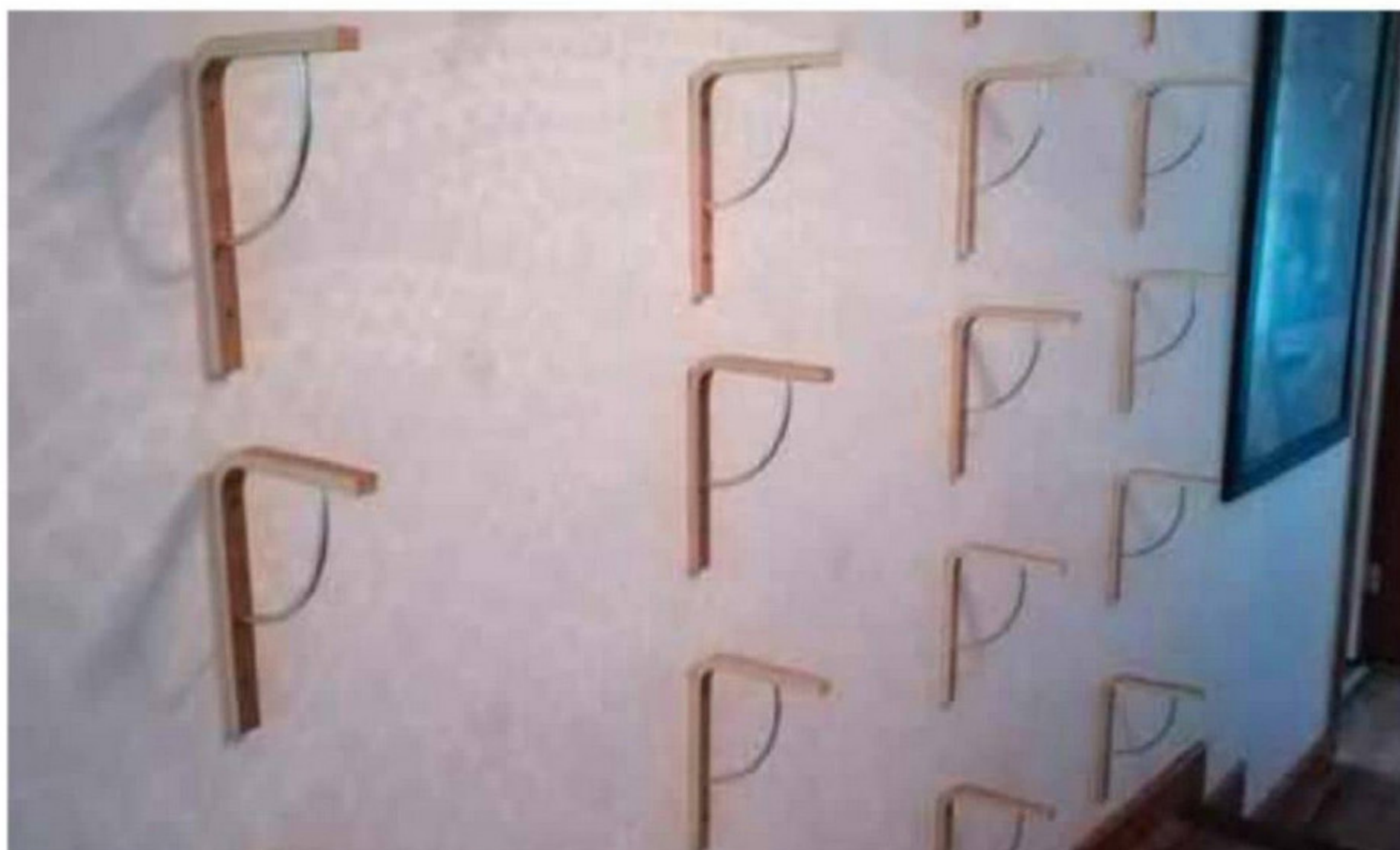
All the brackets in position
