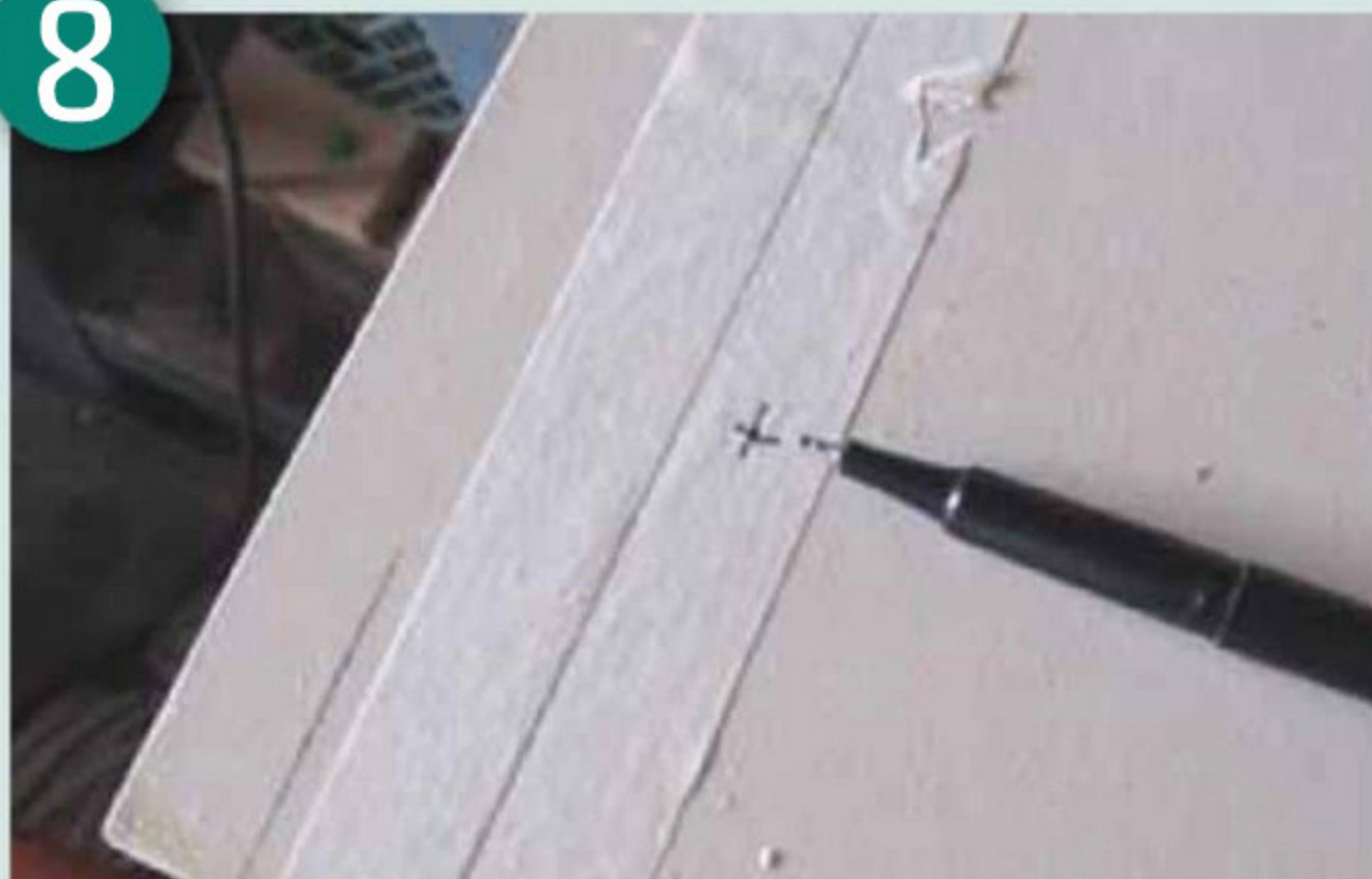
Marking pilot holes for the top
