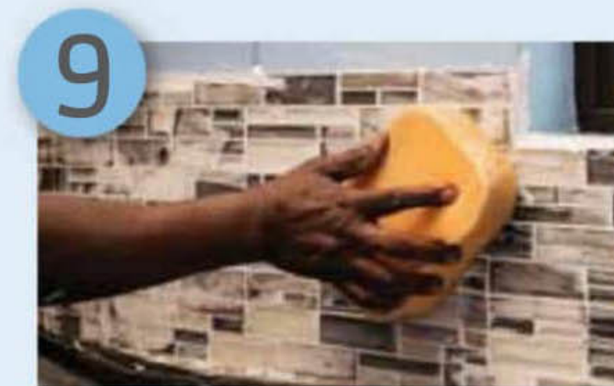
Remove excess adhesive with a damp grout sponge
