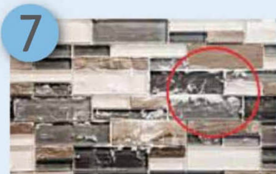
Allow adhesive to squeeze through to form the grout
