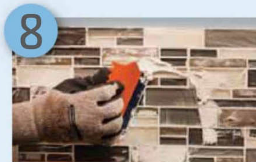
Where necessary, fill in any low areas in the grout joints with extra adhesive
