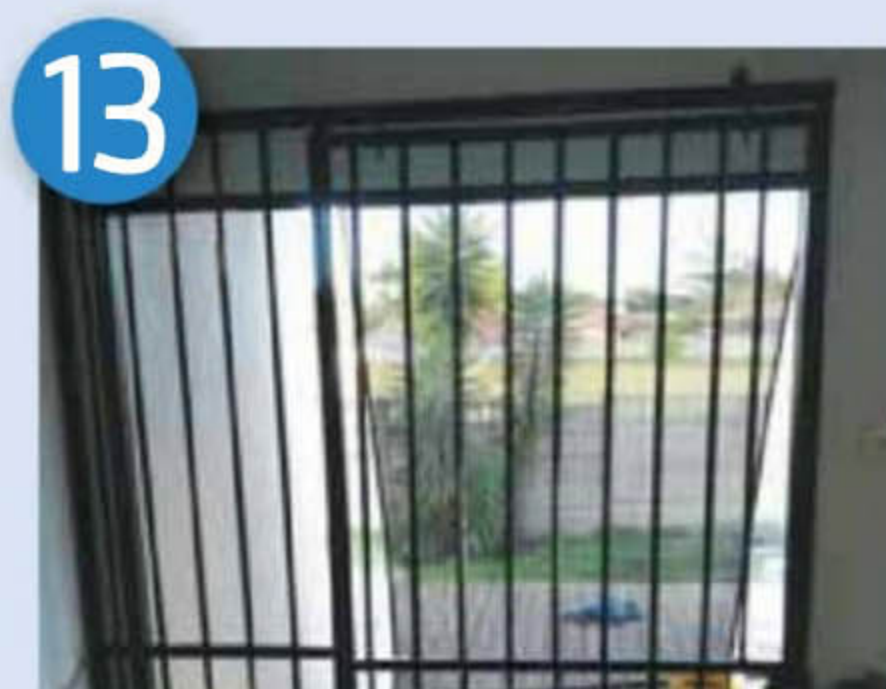
Finished gate in position
