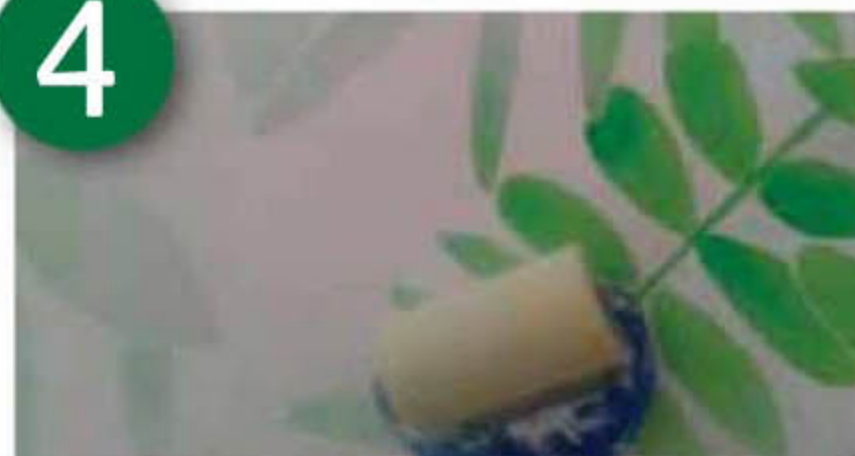
Applying the white background with a roller
