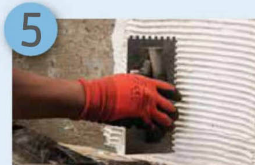
Apply adhesive with a wall trowel
