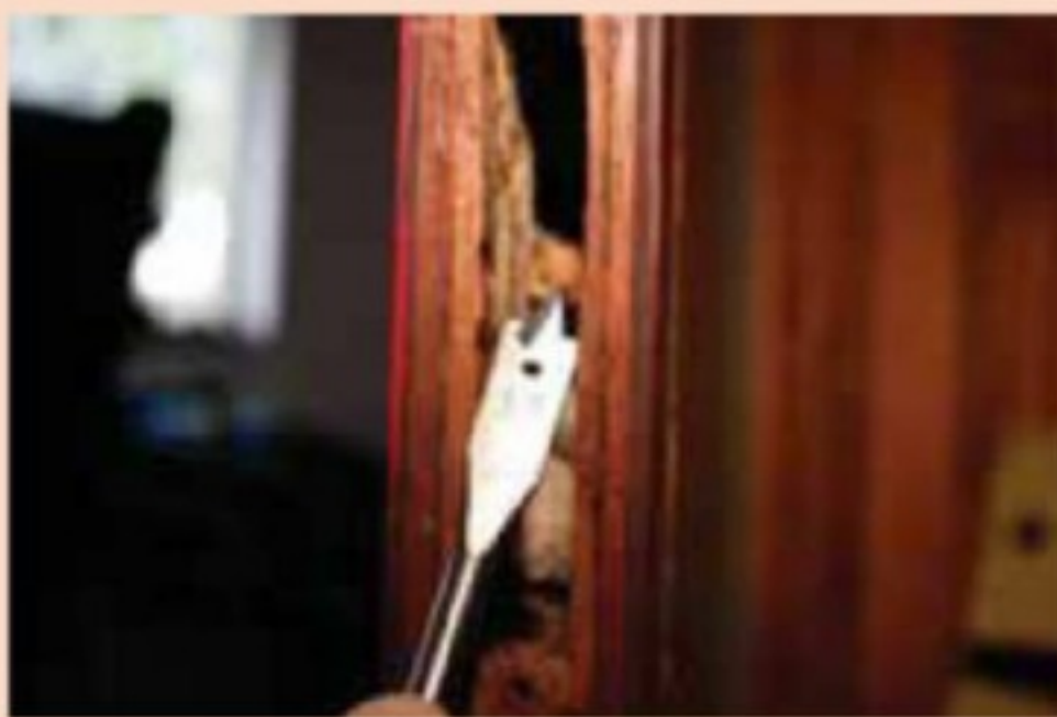
An auger bit is used to make the recess space for the locking mechanism
