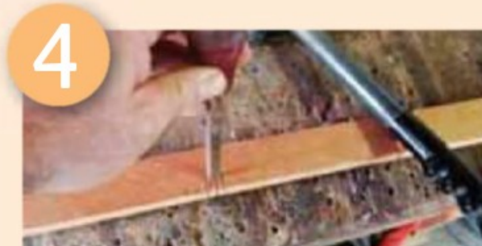
Chisel out notches for burglar guards
