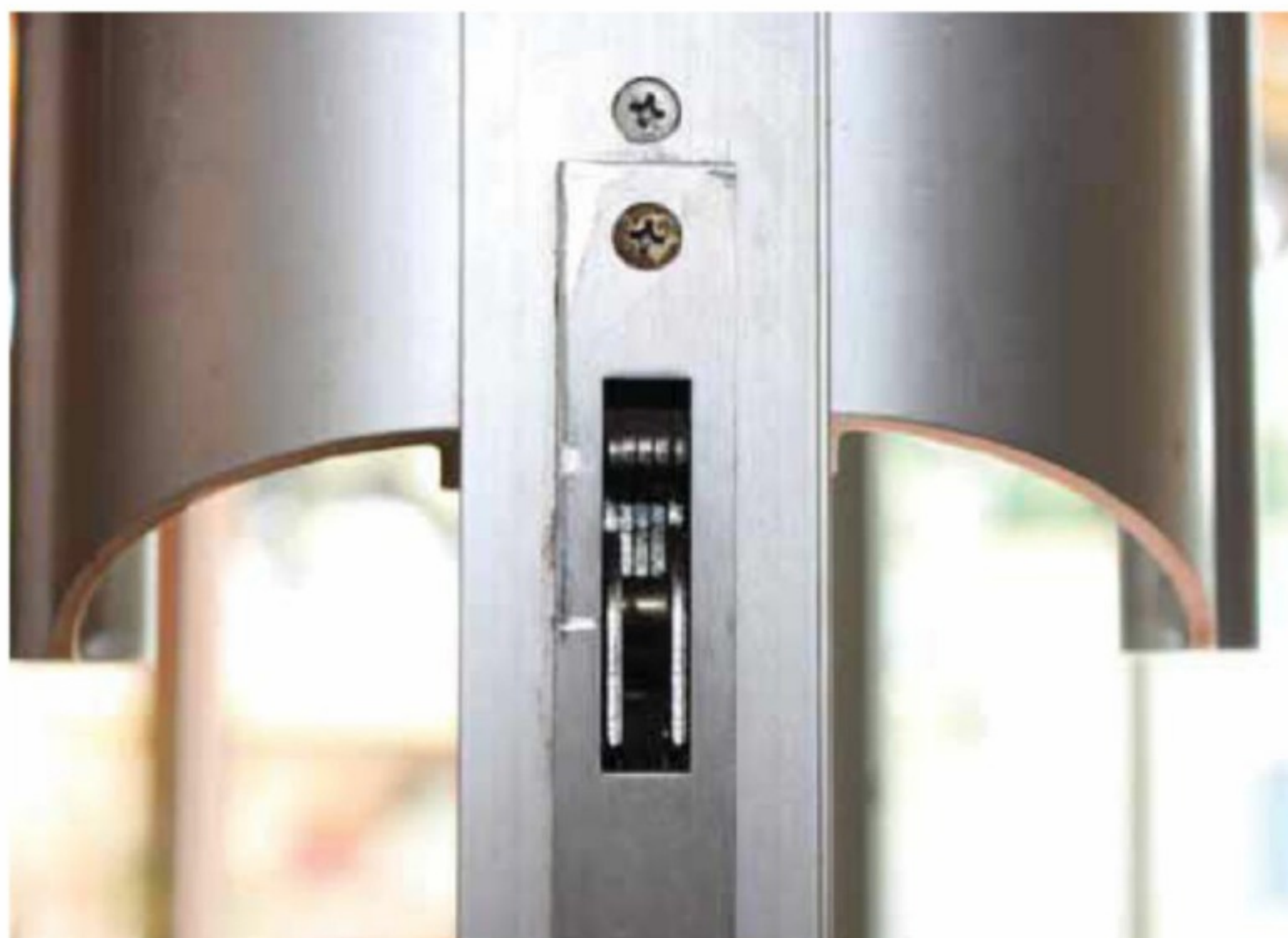
Locking mechanism for an aluminium sliding door
