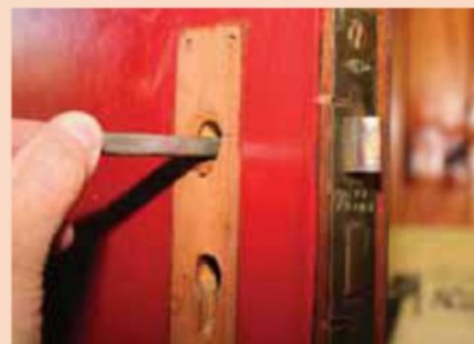
Fitting the spindle for the door handles
