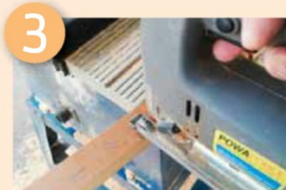
Cut notches with a jigsaw
