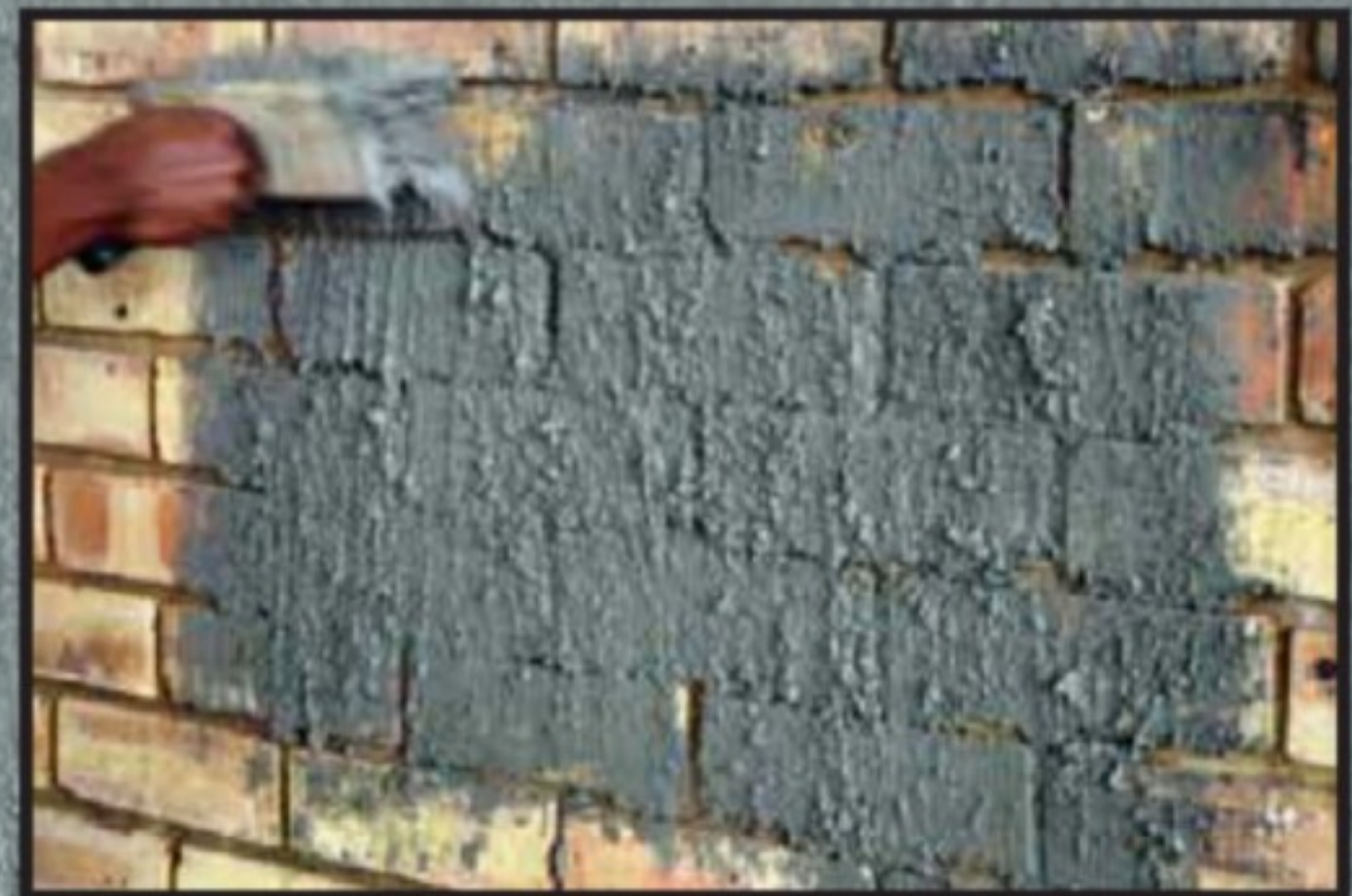
Apply slurry with a block brush - EASY!
