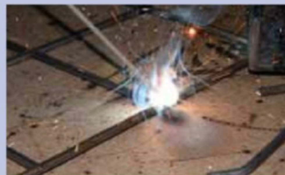
Welding thin round bar
