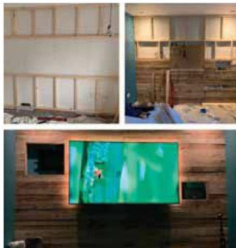
The step-by-step process showing the frame
