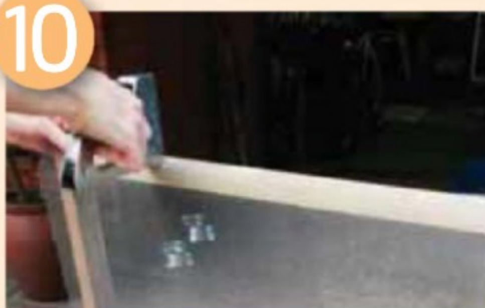
Staple mesh to the frame
