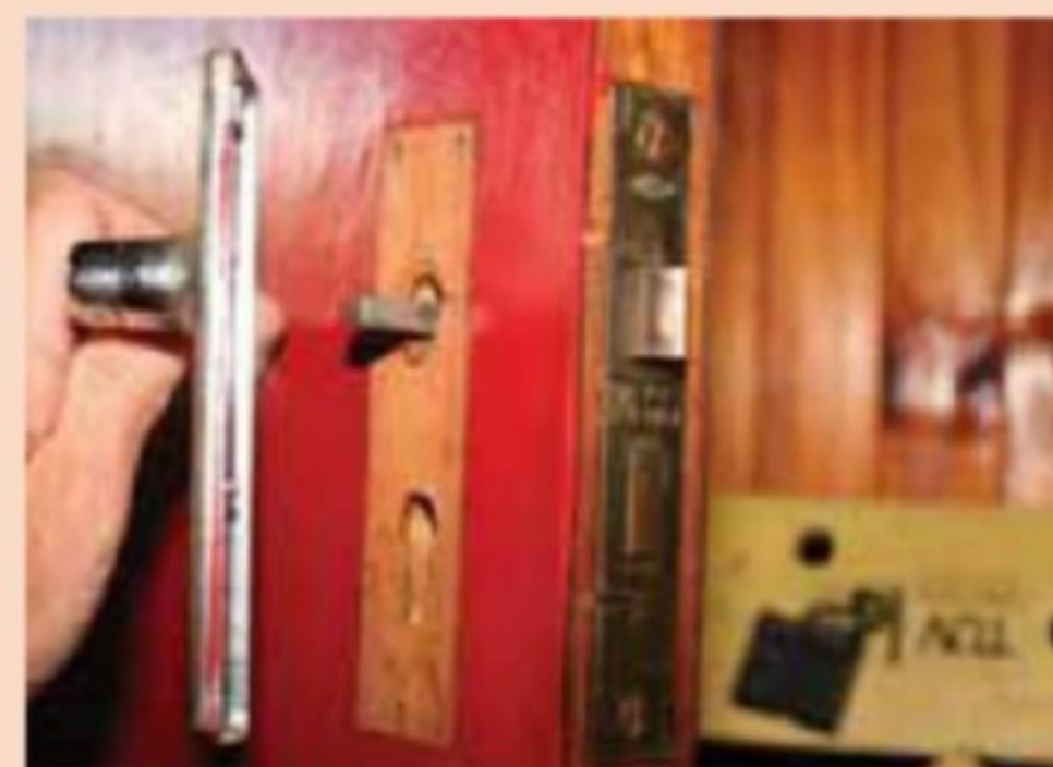
Lastly, the handles are screwed into place
