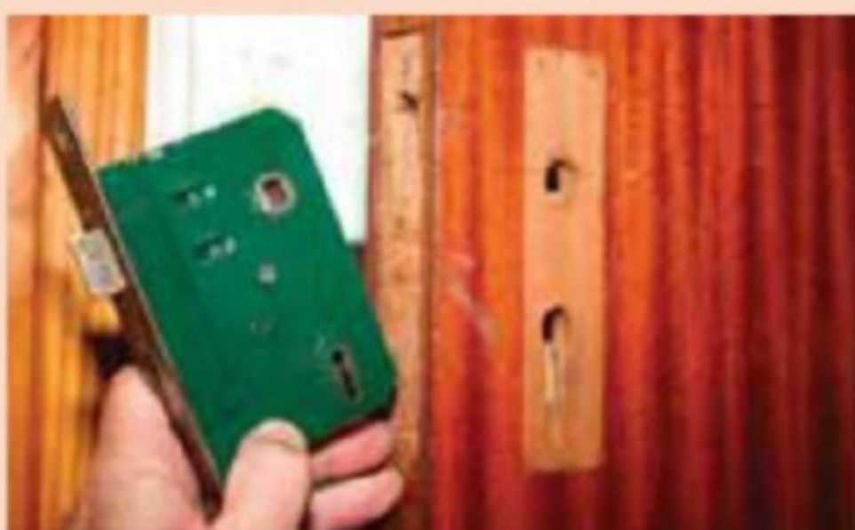
Fitting the locking mechanism
