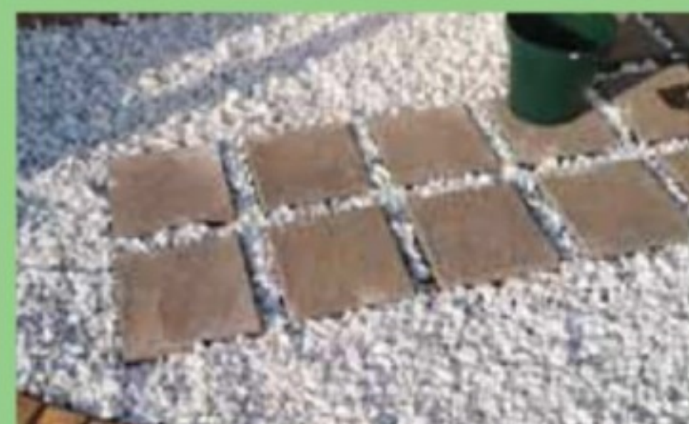
Once the pavers are in, start adding the pebbles
