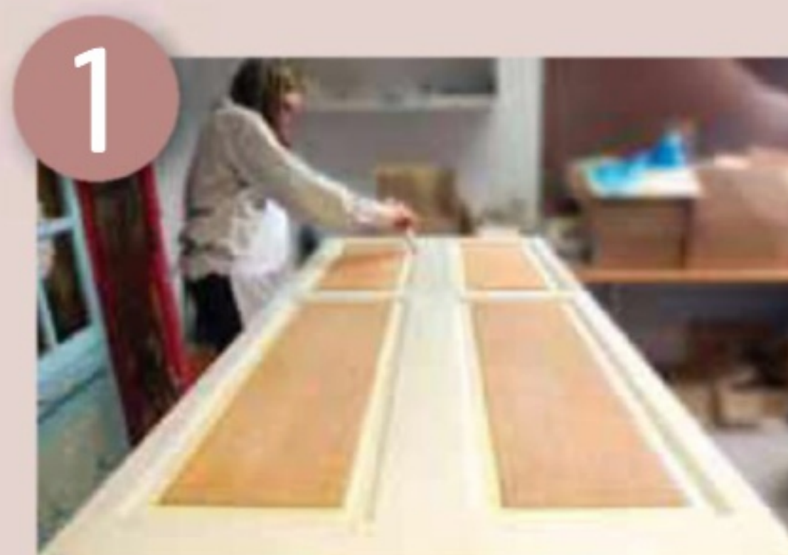
Priming around the panels
