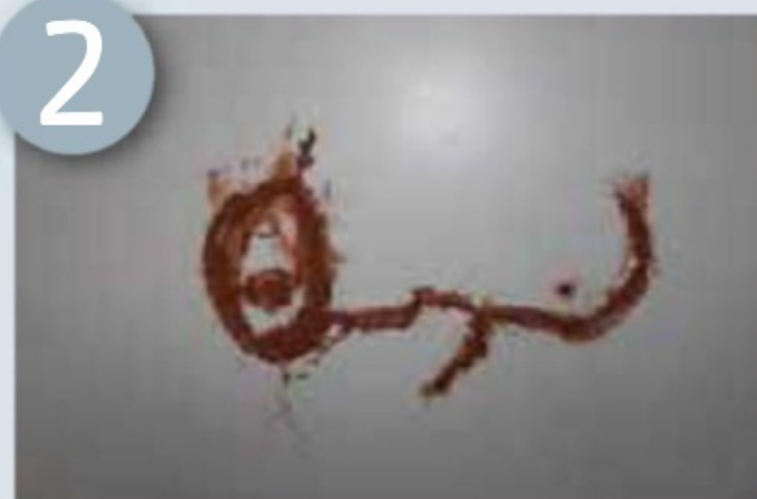
2 Use wood filler to level the repair
