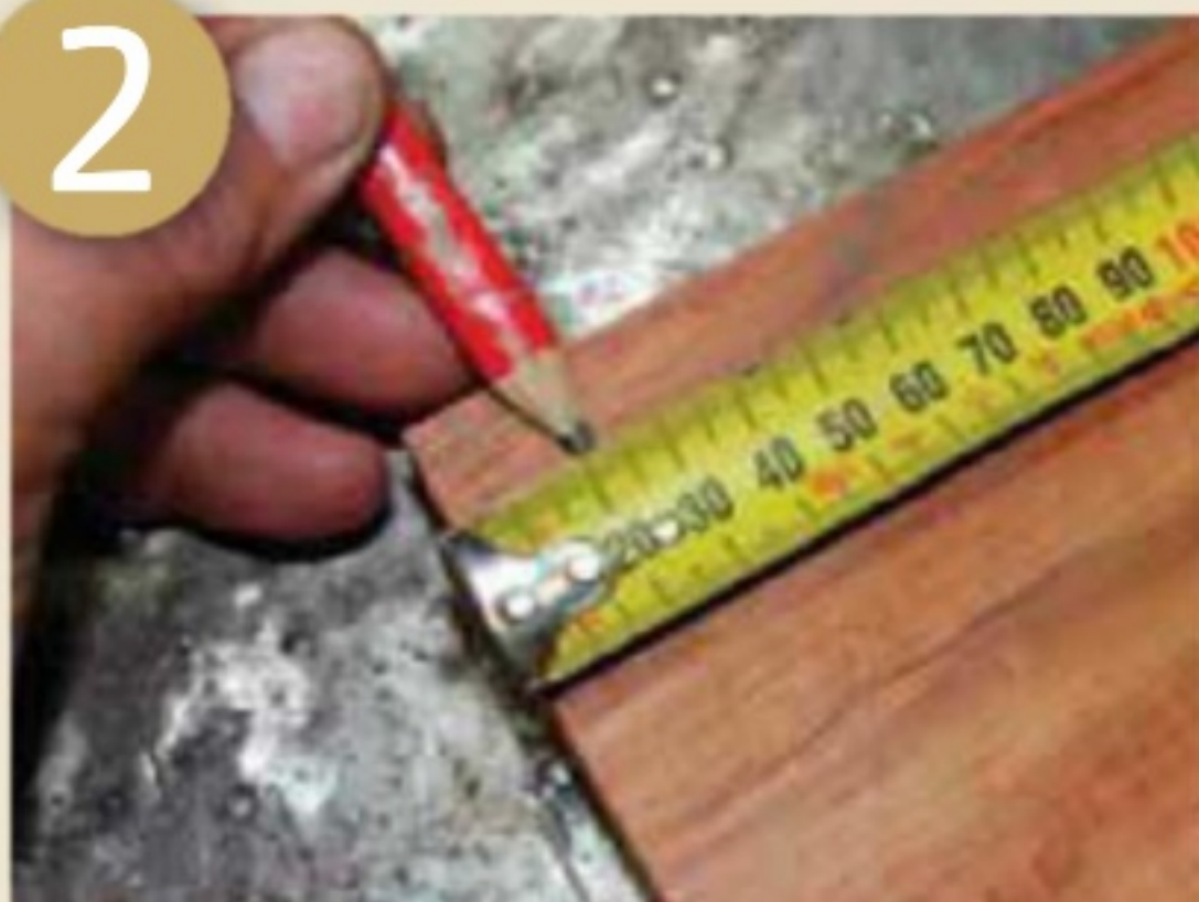
Measure for the pilot holes
