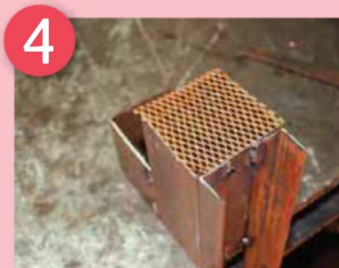
Cut some mesh for the grill
