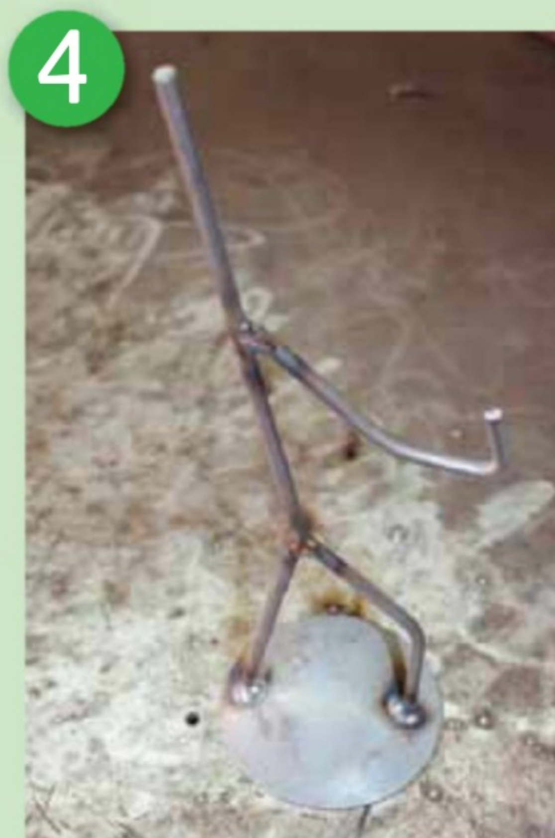
Weld the second arm in place
