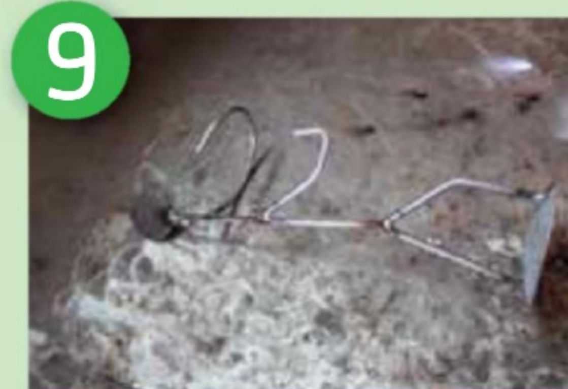
The project before spraying
