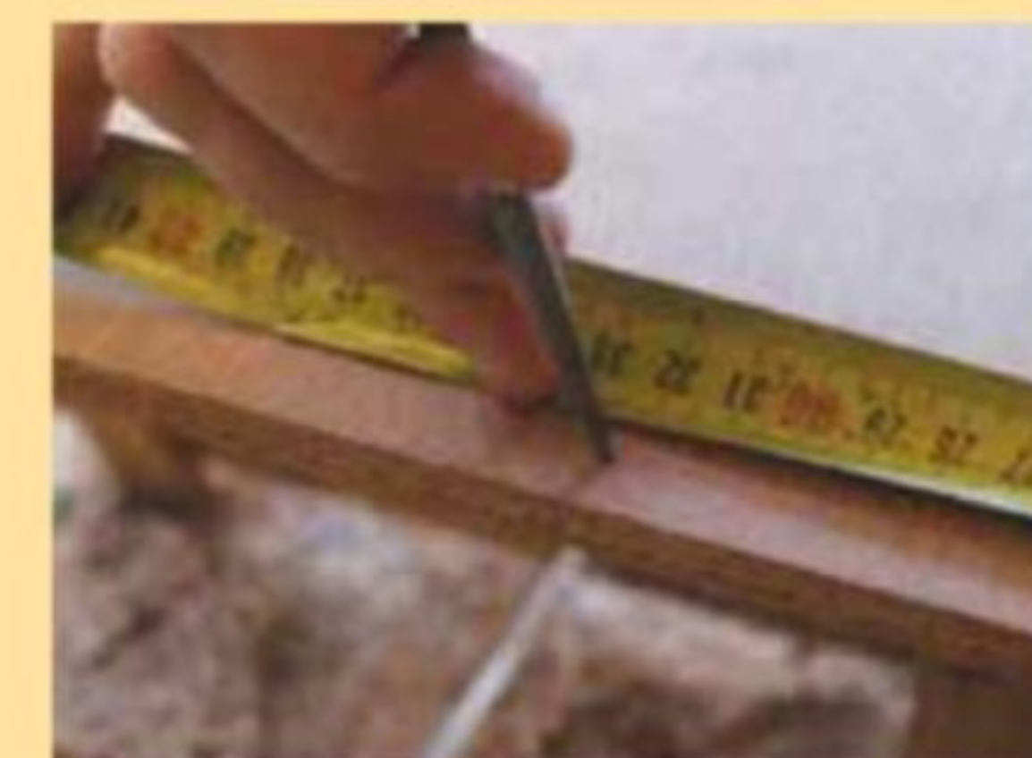
Use an awl and mark the spots to drill pilot holes before nailing and gluing the panels
