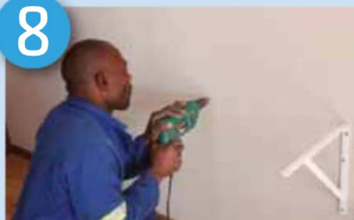
Fit the brackets for the desk
