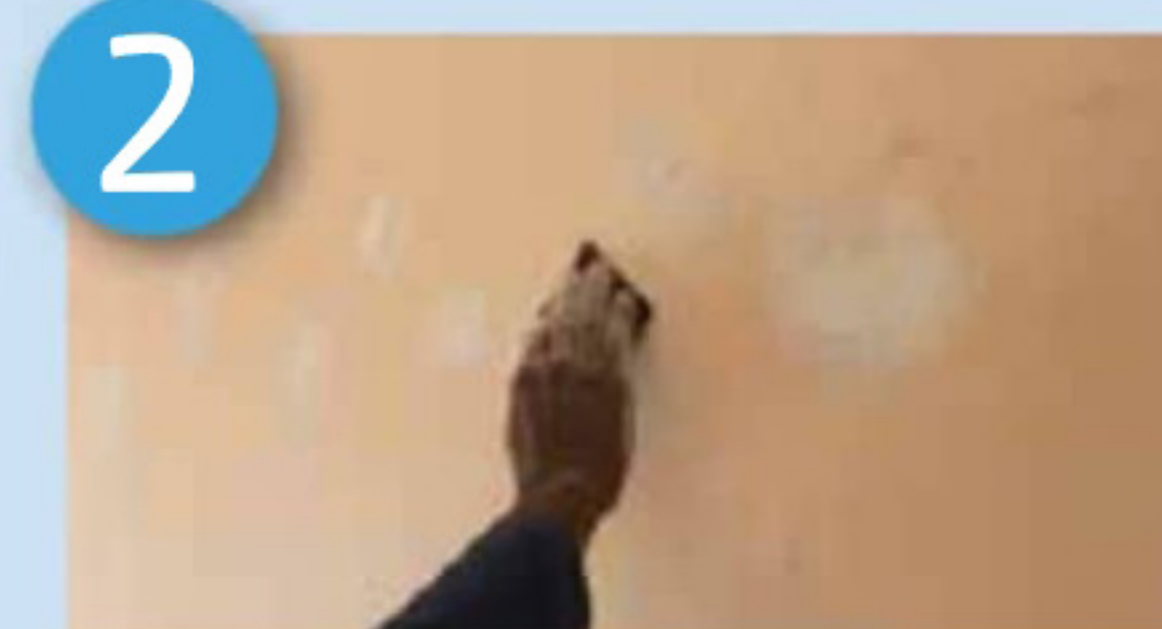
Apply Polyfilla and allow to dry before sanding
