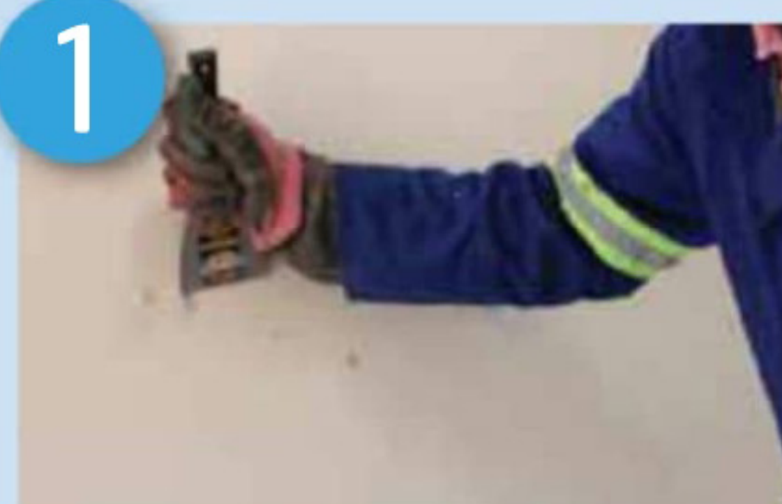
Chip away any holes/cracks
