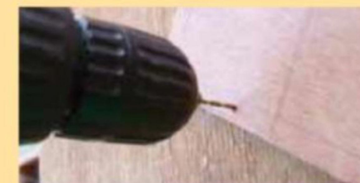
Drill the pilot holes
