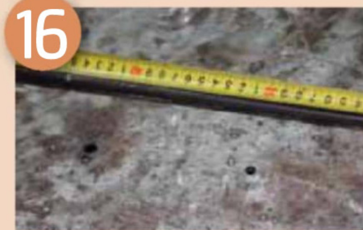
16 Measure 450mm on 8mm round bar
