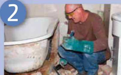
Always wear the appropriate safety gear when working – in this case sturdy gloves and eye protection to protect the eyes from flying concrete chips
