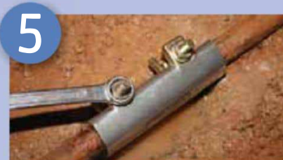
A cascade clamp can be used to seal the leaking pipe as a temporary measure
