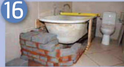
Fitting the bathtub in place to check that everything is in alignment
