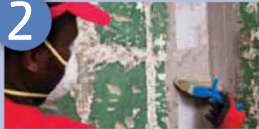
Apply the first coat of waterproofing compound
