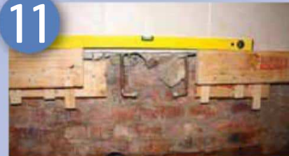
Throughout the installation, make sure that everything is level. This will benefit the installation process later
