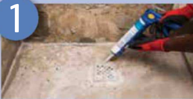
To allow for movement, apply a 10mm silicone bead
