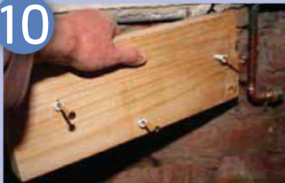
Fitting the timber support beams on the two sides which will support the bathtub at the correct level
