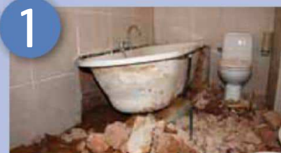
Breaking out the bath to access the plumbing pipes
