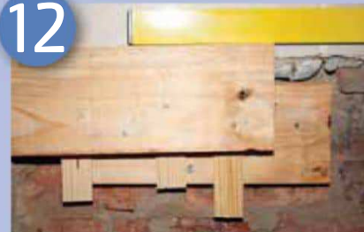
The timber support beams screwed and nailed in position
