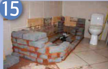
Start of the surrounding brickwork
