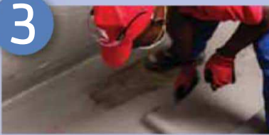
Apply a coat of TAL Sureproof over the walls and floors not covered by the membrane
