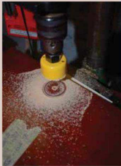
The hole for the power cables
