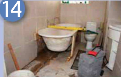
Measuring and levelling the bath
