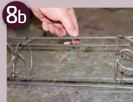
Weld the scrolls in place
