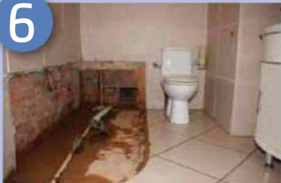
Complete removal of the bath
