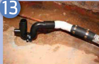
Fitting the rubber bath trap and 50mm PVC pipe with 45° elbow bend
