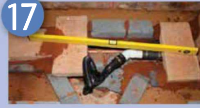
Concrete blocks were placed beneath the bathtub to protect the pipework below and the cavity filled with river sand
