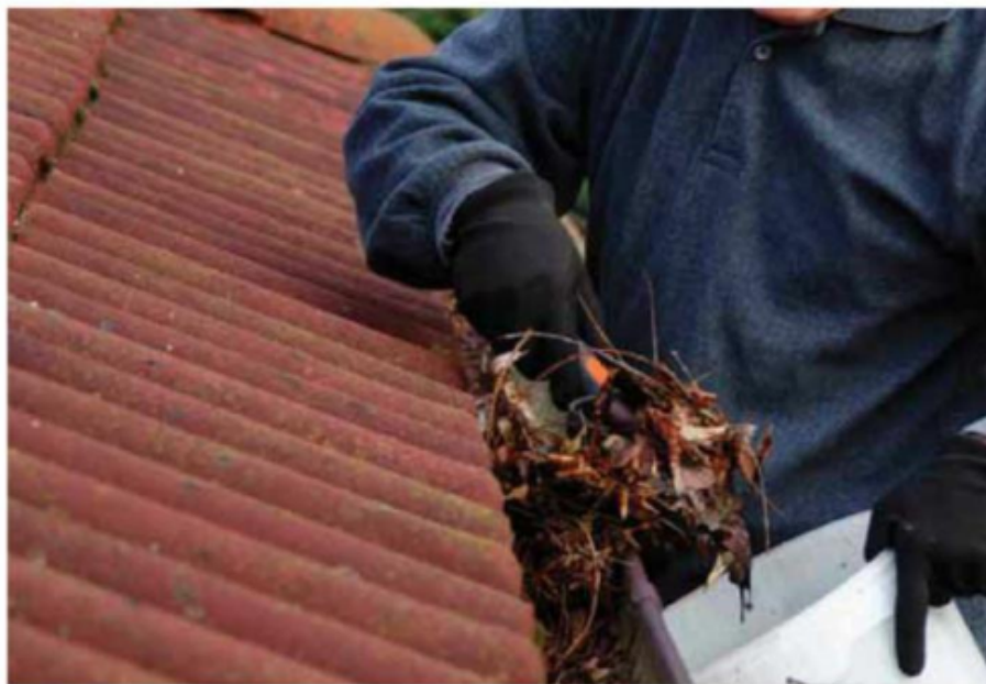
It is imperative that gutters are kept free of leaves, twigs and sand which could cause a blockage
