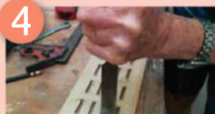
A sharp chisel comes in handy to open the windows
