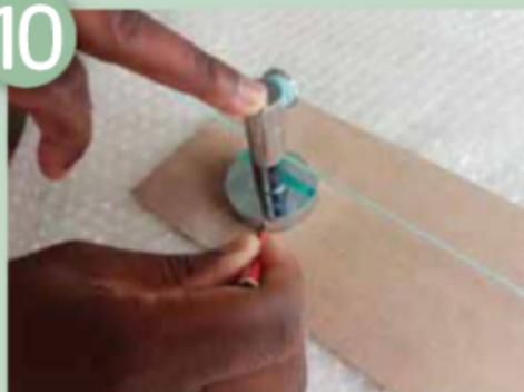
Marking out the shelf template
