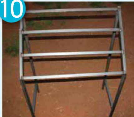
Weld all cross beams in place
