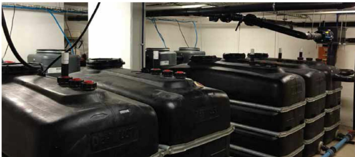
This commercial system recycles 12 kilolitres of water daily. Pic: Akwasolv
