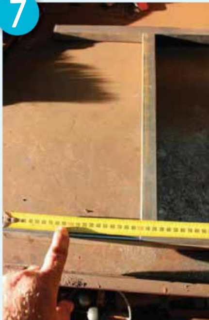
Measure 200mm from bottom
