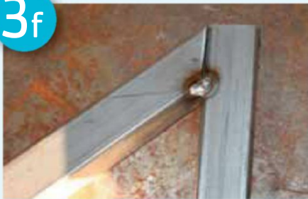
Weld in place
