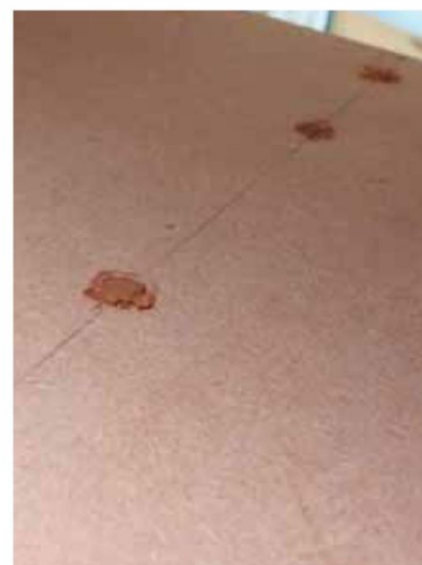
The countersunk screws can be filled in with dowels cut to size or wood filler
