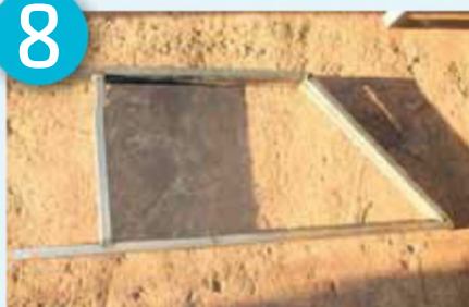
Weld cross braces in place
