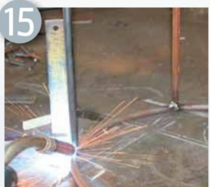
Weld legs in place
