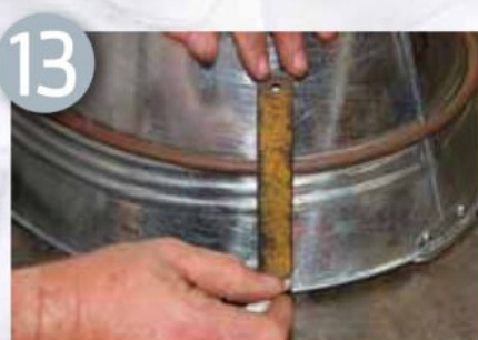
Use a square to trace line up
