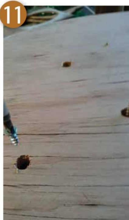
Four holes done
