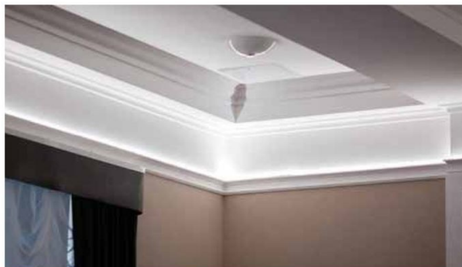
LED cornices have a slot for LED up- or downlights to create ambient lighting in the room
