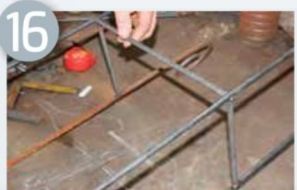
Weld support in place
