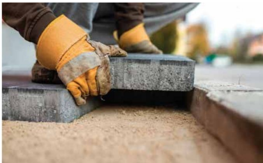
Before laying your pavers, prepare a base layer, using intermediate grain river sand
