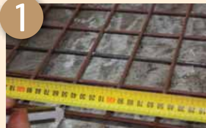
Measure and cut components to size
