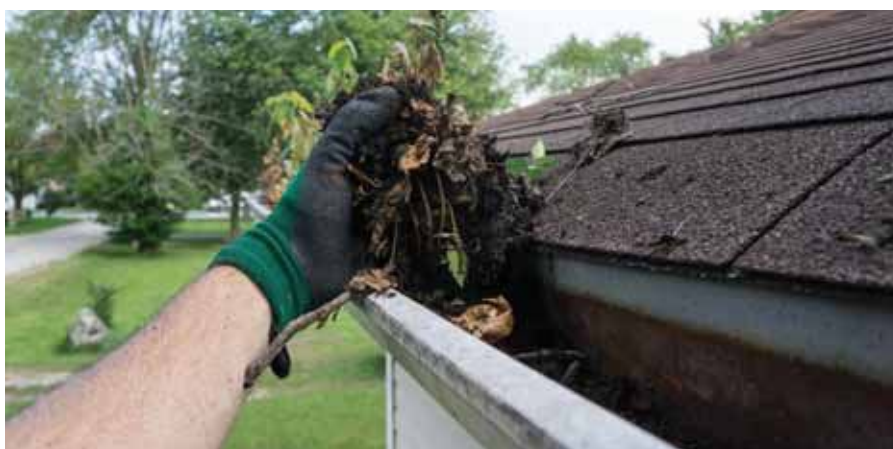
Remove debris from guttering
