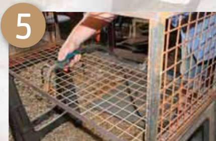
Tack weld mesh in place
