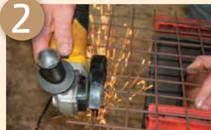
Cut the mesh to size
