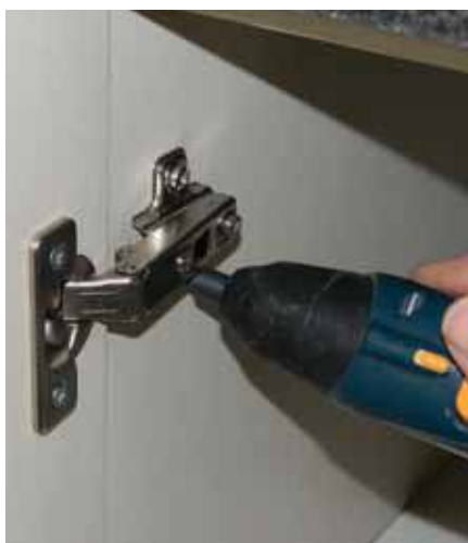
Check all cupboard hinges and tighten up where necessary
