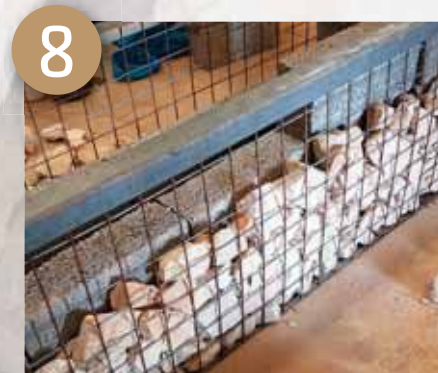
Place bricks on the inside
