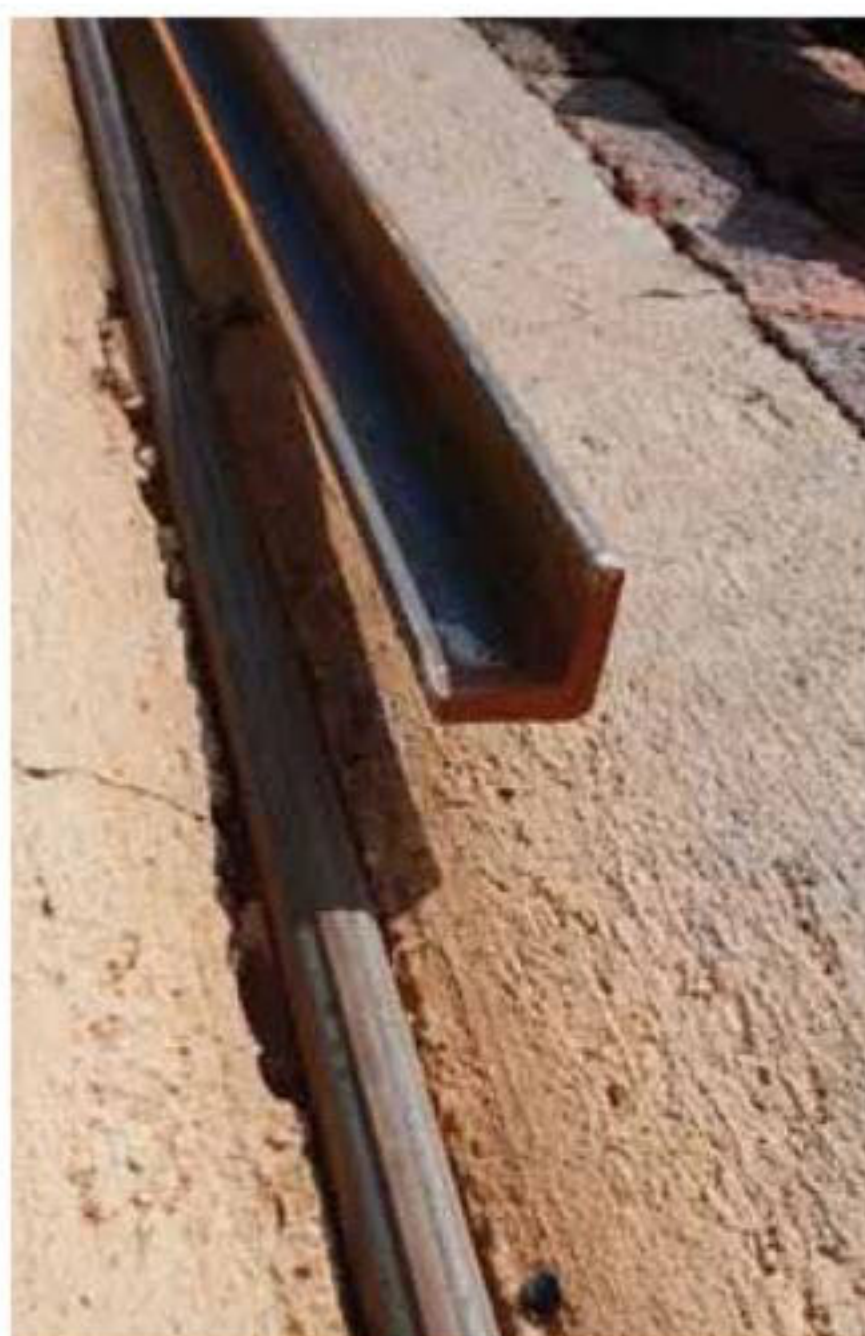
The new track on the old track
