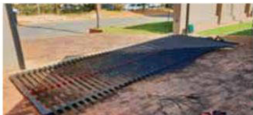
Original gate is removed
