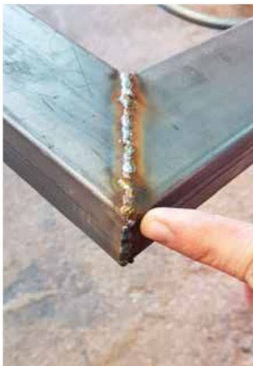
Weld the top frame
