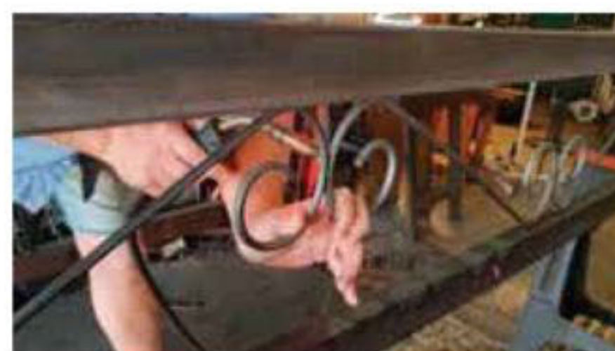
Weld scrolls in place
