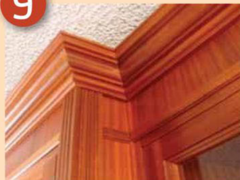
Completed crown moulding
