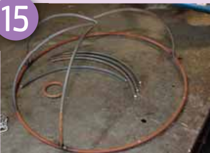
Weld up the curved sections
