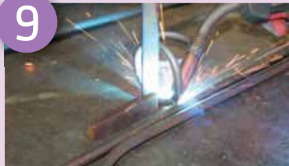
Weld rings in place
