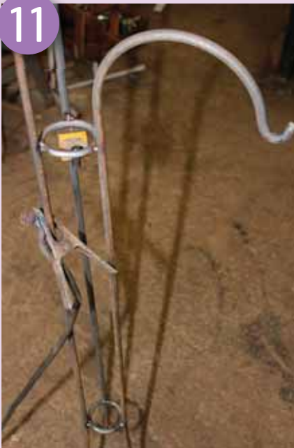
Weld rings in place
