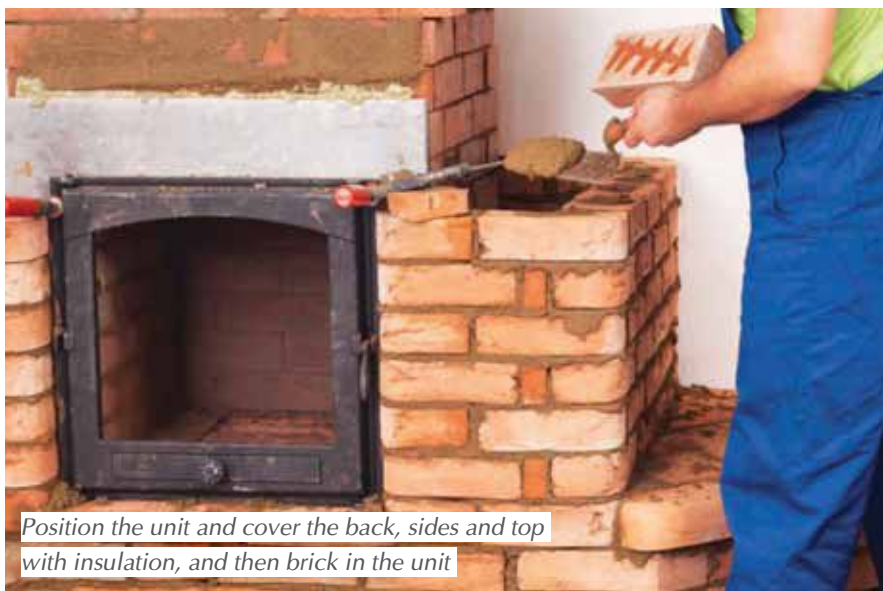
Construct brick support walls for the unit to your desired height
