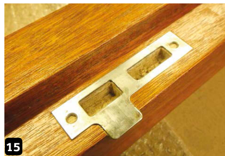
The striker plate fitted
