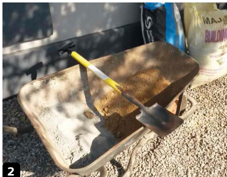
2 The concrete we used had to be mixed with two parts building sand
