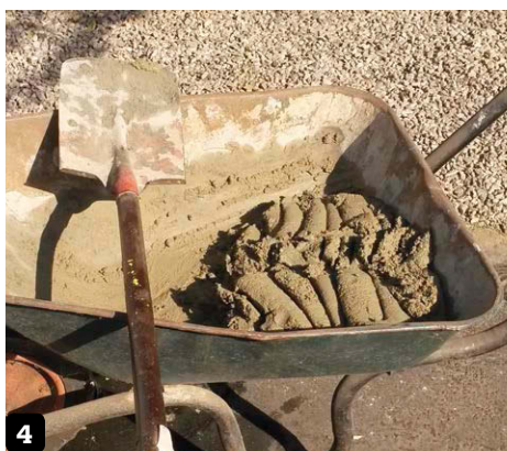
4 A wheelbarrow comes in handy when mixing a small amount of cement
