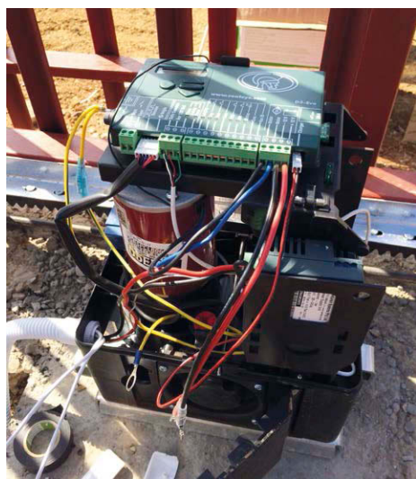
Terminate the wiring and complete setup of the gate parameters
