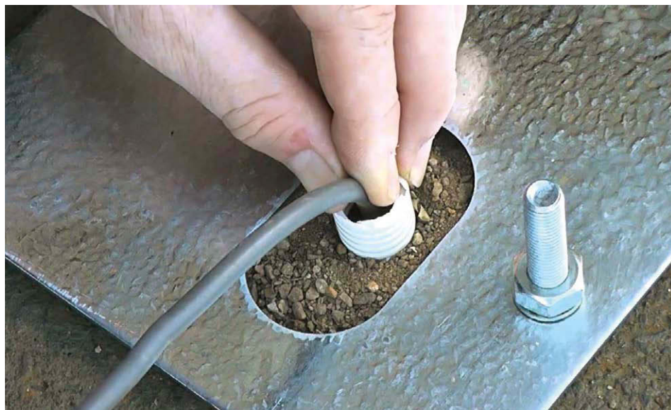
Consider your wiring before securing the base plate
