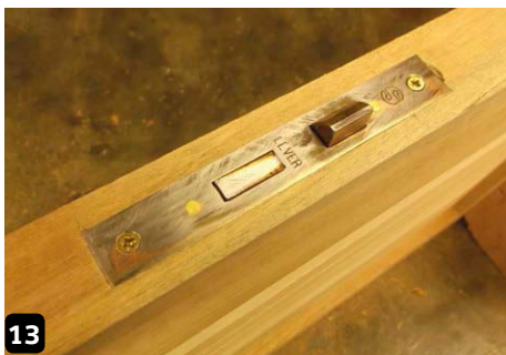
The lock fitted
