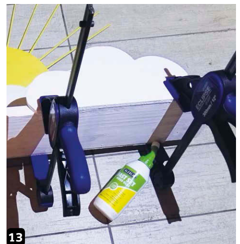
The cloud in front was glued to the front of the shelf with glue only
