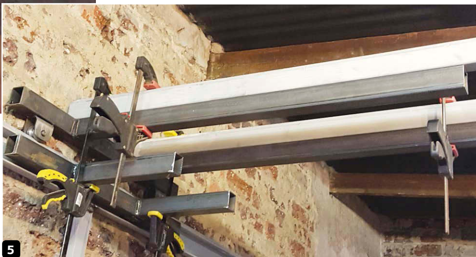
5 Careful measurements were taken to ensure the end truck guide rails ran true with the runway beams
