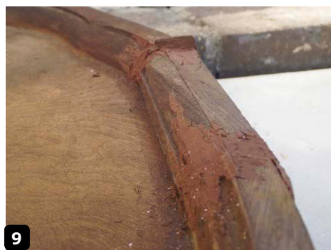
9 Gaps in-between the inserts were filled with wood shims and wood filler
