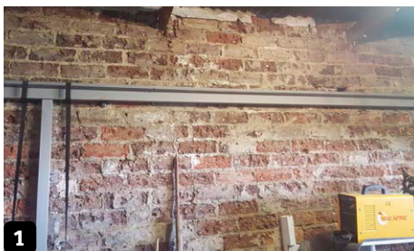
The pillars and runway beams were fixed to the walls of the workshop with rawl bolts
