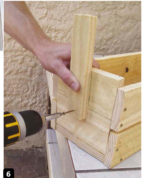
6 The supports for the handle are screwed to the side of the box
