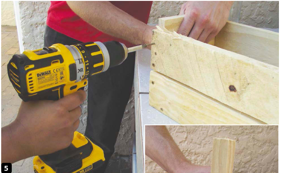
5 Aarifah screwing the uppermost slat in place
