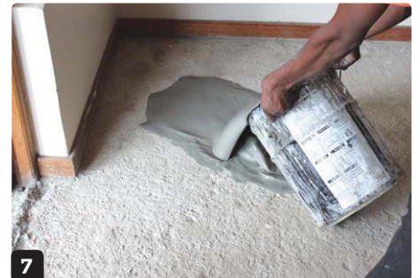
6 Mix the self-levelling compound well
