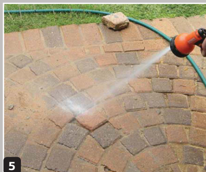
Clean away excess using a hose set on medium spray
