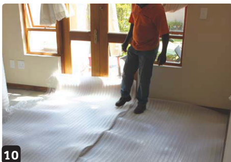
10 Lay the plastic underlay
