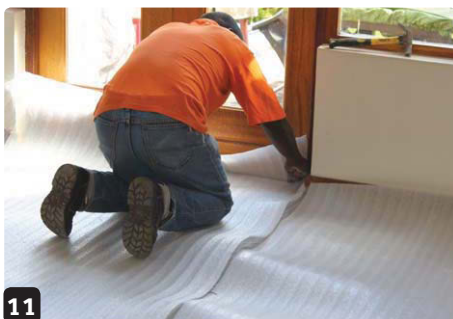
11 Use a sharp knife to cut the underlay
