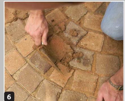
Re-grout the new paver and allow to dry completely
