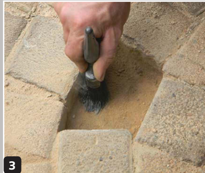
Remove any sand or debris from the cavity or the new paver may not be level
