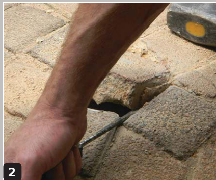
Once the paver starts to loosen, it is easy to lift with a screwdriver
