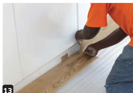
13 You should leave a 10mm clearance along each wall
