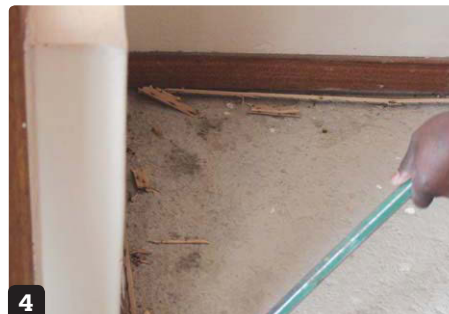
3 Everything comes out down to the raw concrete floor
