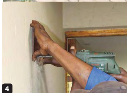
4 Drilling straight and level in the right spot is essential
