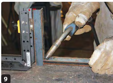
9 Weld the 200mm angle iron pieces onto the outer ends of the 470mm length of angle iron
