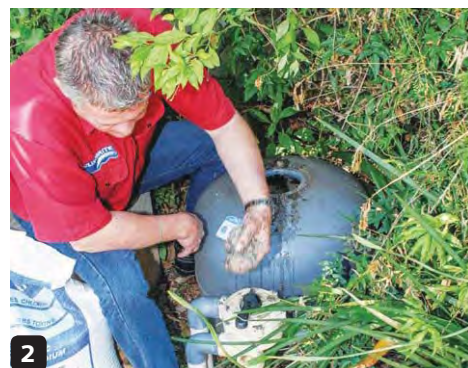
2 Remove the old filter sand
