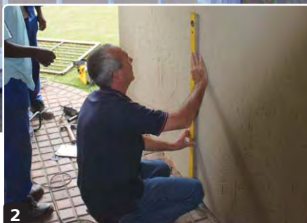
2 Measuring and marking is of vital importance – get a helper to hold the gate in place and examine the placement
