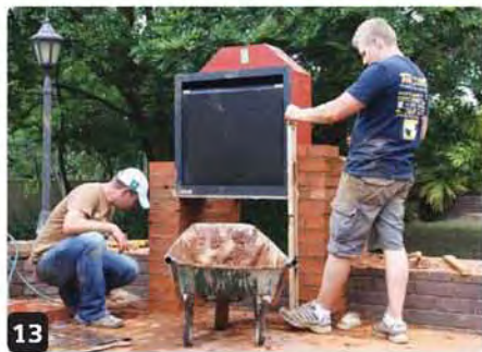
12 Three lintels are necessary for this braai, plus another one on which to build the back wall
