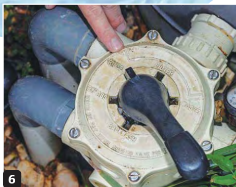
6 After the five-minute backwash cycle, set the pump valve to 'rinse' for two minutes
