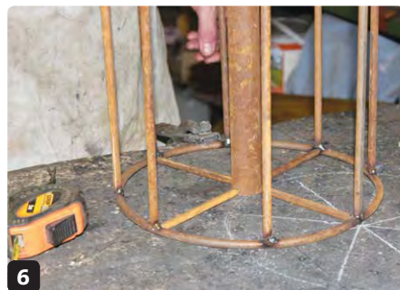
6 Weld the short pieces of round bar onto the outer rings
