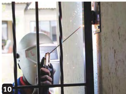
10 Weld the bottom hinge to the gate and to the wall plates and then the top hinge
