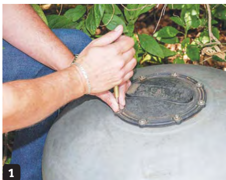
1 Remove the filter lid
