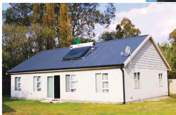
▲ This home was constructed using Structural Insulated Panels – they consist of an insulating foam core sandwiched between two facings
