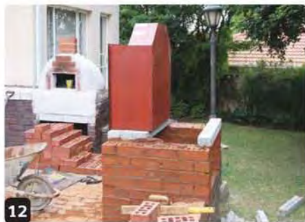
12 Three lintels are necessary for this braai, plus another one on which to build the back wall
