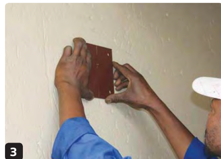
3 Mark the top plate onto which the hinges will be welded
