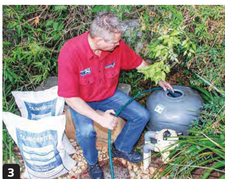
3 Fill the tank halfway with tap water
