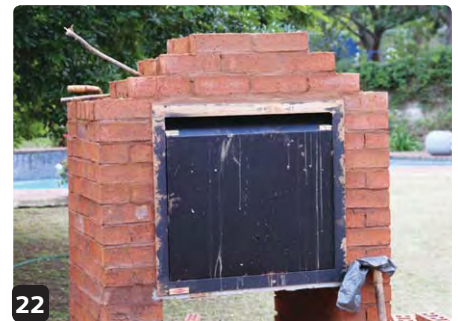
20 A stick held the space for the light fitting wire
