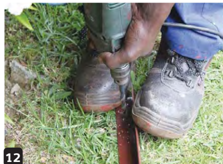
12 Drill holes through the angle iron so that it can be secured to the wall
