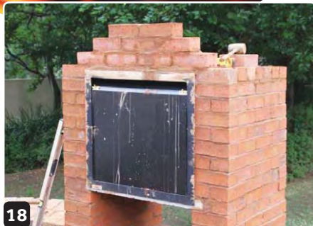
15 You do not have to fill the holes in the bricks
