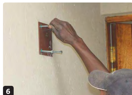
6 We used 8mm x 75mm coach screws with plugs
