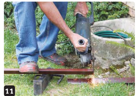
11 Cut the angle iron to size
