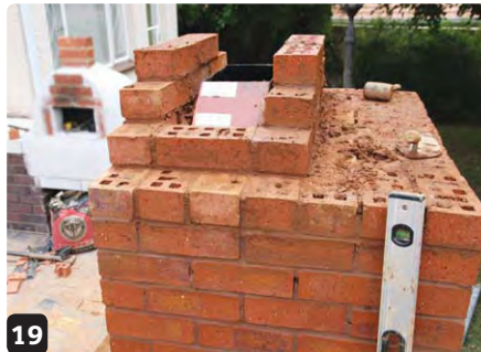
16 A perfect level at the top of the structure
