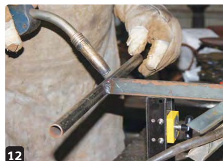
12 Weld a piece of pipe onto the other end of the 700mm angle iron to serve as a handle
