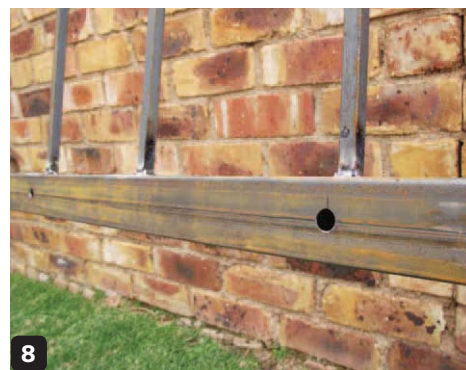
Drill 12mm holes in the 1 560mm square tubing of the headboard
