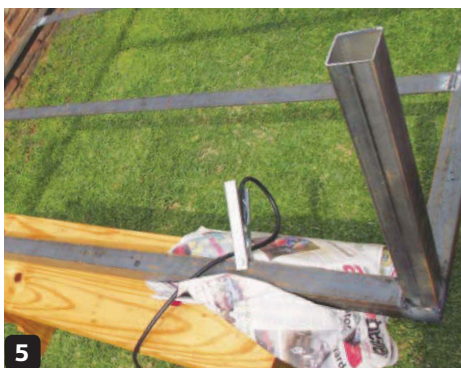
Weld both the square tubing legs onto the underside of the base's frame
