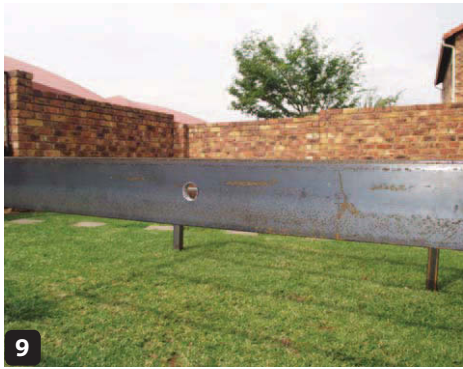
9 Line up the frame and the headboard with each other and transfer the holes in the headboard onto the frame and drill them as well
