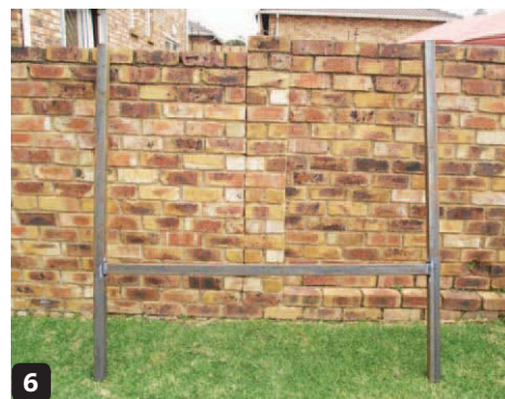
Construct an H-shape from the two 1 600mm lengths and one 1 560mm length of square tubing. The horizontal length is 500mm from the bottom
