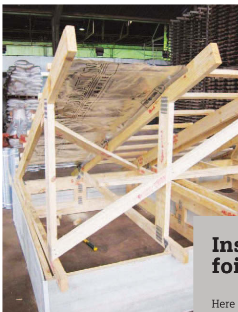
▲ RadenShield ClimaGuard is a DIY friendly system whereby the reflective aluminium sheets are stapled to the inside of the roof rafters.
