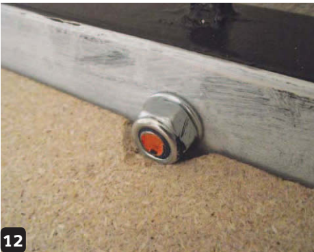
12 To enable the wood to go in, you might have to cut a slot so that the wood can fit underneath the nut
