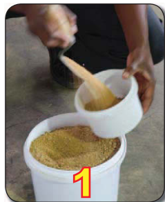
Measure Plaster Sand
