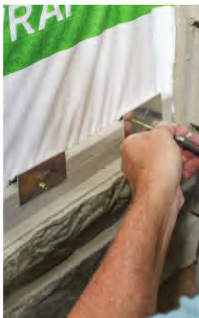
▲ Install the BellaStone panels using 2-1/2-in. corrosion-resistant screws and metal clips provided by the manufacturer.
