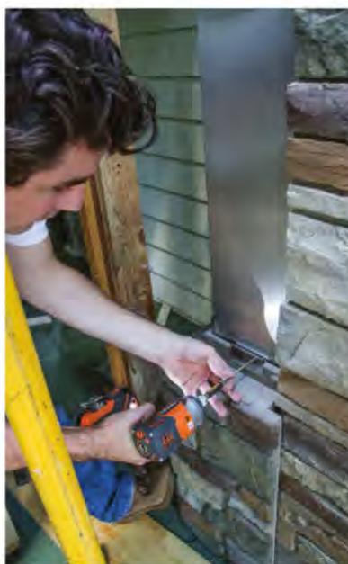
▲ After installing the panels, attach the BellaStone Quoin Corners along the outside corners of the chimney chase.
