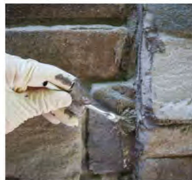
▲ Caulk all joints and seams to prevent water intrusion; then apply stone dust to the caulk with a small brush.
