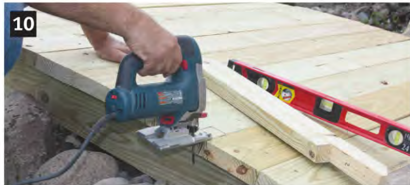
▲ Tip: By angling the base of the jigsaw so the blade is plumb, you can easily cut the angled notches in the deck boards.
