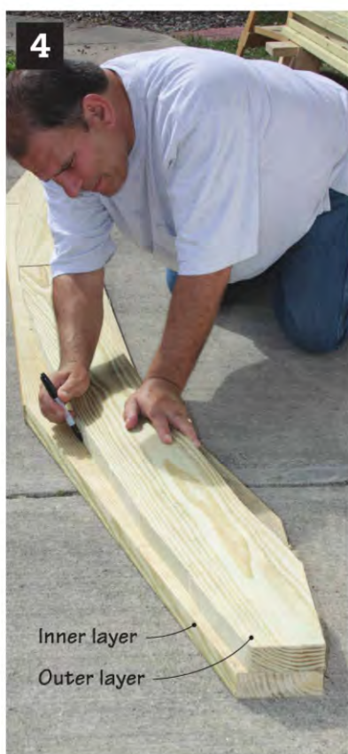
▲ Trace the curves from the outer layer onto the inner layer.
