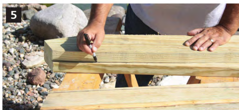
▲ Use the previously cut beam sections as templates to trace the curves on all identical beam sections.
