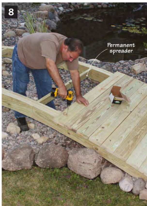
▲ Fasten the deck boards in place with two 3-in. deck screws at each end, maintaining a 2-in. overhang on both sides.
