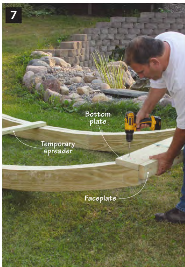
▲ Flip the beams upside down to attach the bottom plates.
