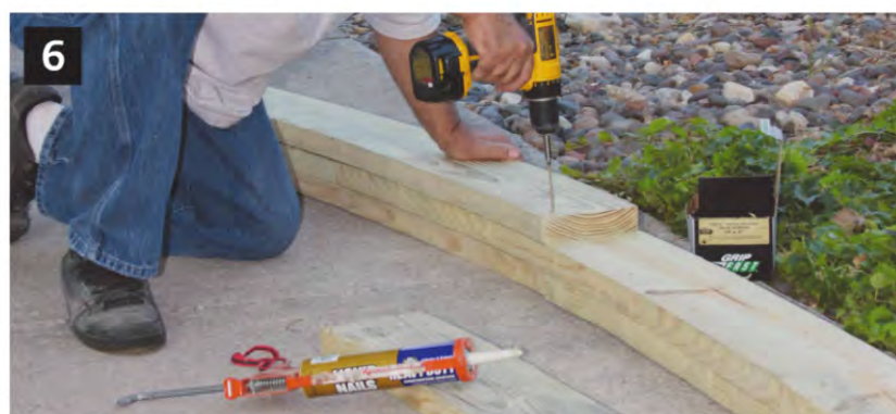
▲ Glue and screw together one inner layer and two outer layers to make the arched beams. Use construction adhesive and 2-1/2-in. or 3-in. deck screws.
