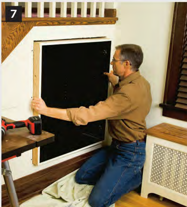
▲ Slide the cabinet into the opening so that the front edge is flush with the outside face of the drywall. Attach the cabinet to the framing with screws.
