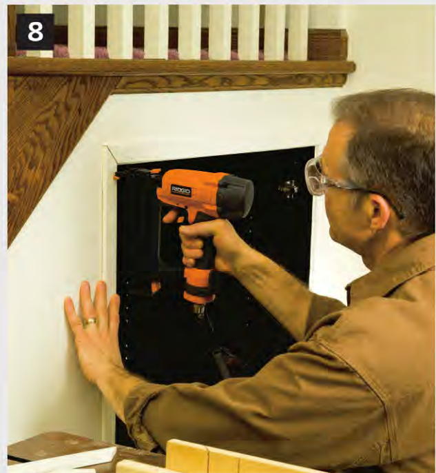
▲ Miter-cut the trim to fit around the cabinet. Attach the trim with 1-1/2-in. brad nails. Then fill the nail holes, touch up the paint and reattach the doors.
