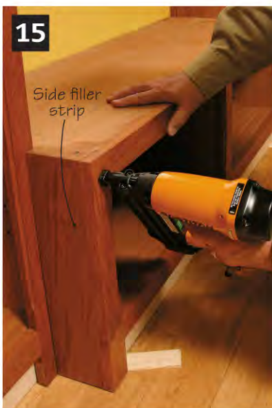
15 ▲ Solid filler strips conceal the sides of the window-seat cabinet. The window seat face frame is fastened with 2-in. finish nails.
