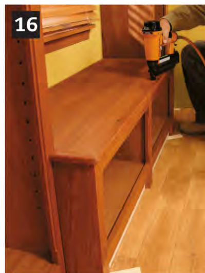
16 ▲ Attach the window-seat board with 2-in. finish nails. To prevent nails from popping through the top of the window-seat cabinet, be careful to drive them into the face frame and cabinet sides.
