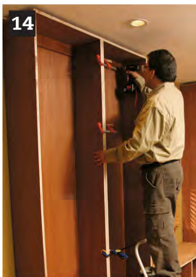
14 ▲ Install the rest of the cabinets. Secure the cabinet sides to each other with 1-1/4-in. screws, to the wall by driving 3-in. screws through the wall cleat, and to the plinth.
