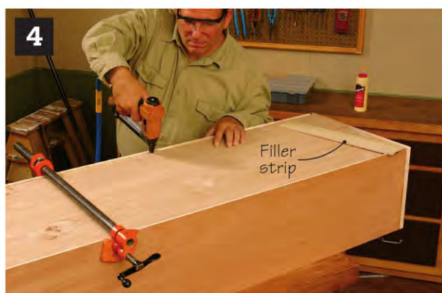
▲ Attach the back panel to the cabinet with glue and 1-in.-crown staples. Then attach a 3-in.-wide strip of the back material to fill the gap left behind the wall cleat.
