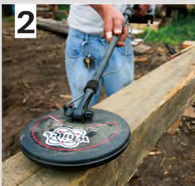
2 ▲ The sawing service then uses a metal detector to locate concealed metal. The metal is removed before machining.
