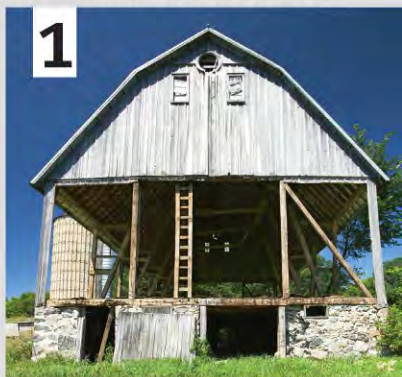
1 ▲ The barn siding and interior fixtures are removed before the frame is knocked down and dismantled.
