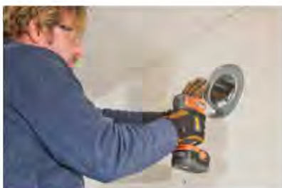
▲ Cut a vent hole and install the vent-pipe thimble.
