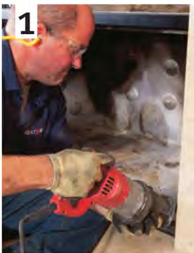
1 ▲ Cutting away parts of the existing fireplace may be necessary to accommodate a new gas insert.
