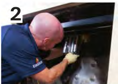
2 ▲ Two flexible pipes run up the existing chimney to provide fresh air and allow exhaust to escape.
