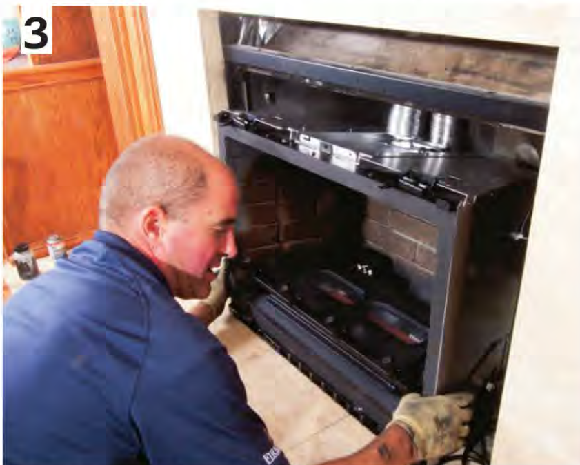
2 ▲ Two flexible pipes run up the existing chimney to provide fresh air and allow exhaust to escape.
