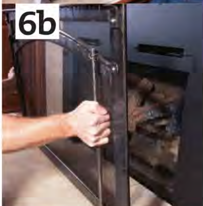
▲ After the logs are in place, a tempered-glass panel is set into the opening to seal the firebox.
