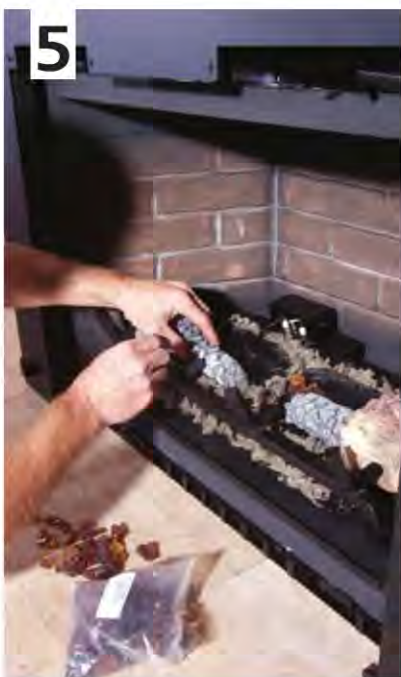
▲ Ember material, glass rock and ceramic logs are carefully placed around the burners.
