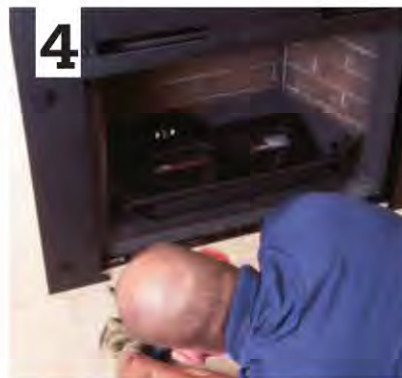
▲ A surround is attached to the insert to cover the open areas around it. The surround also supports a door.
