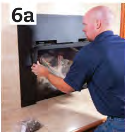
▲ Ember material, glass rock and ceramic logs are carefully placed around the burners.
