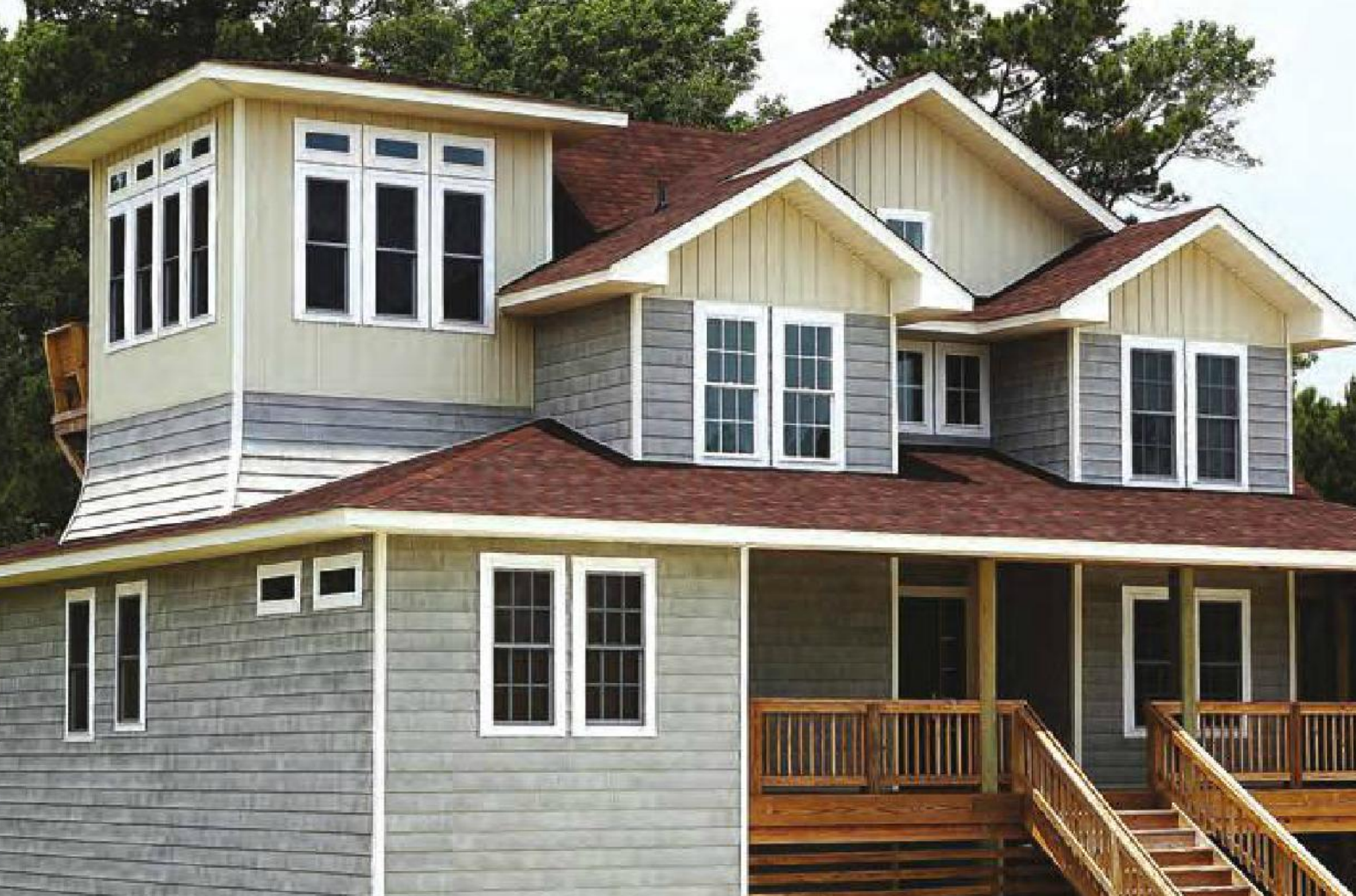
This modern beach cottage combines vertical vinyl siding, straight shakes and window lineals to enhance architectural interest.
