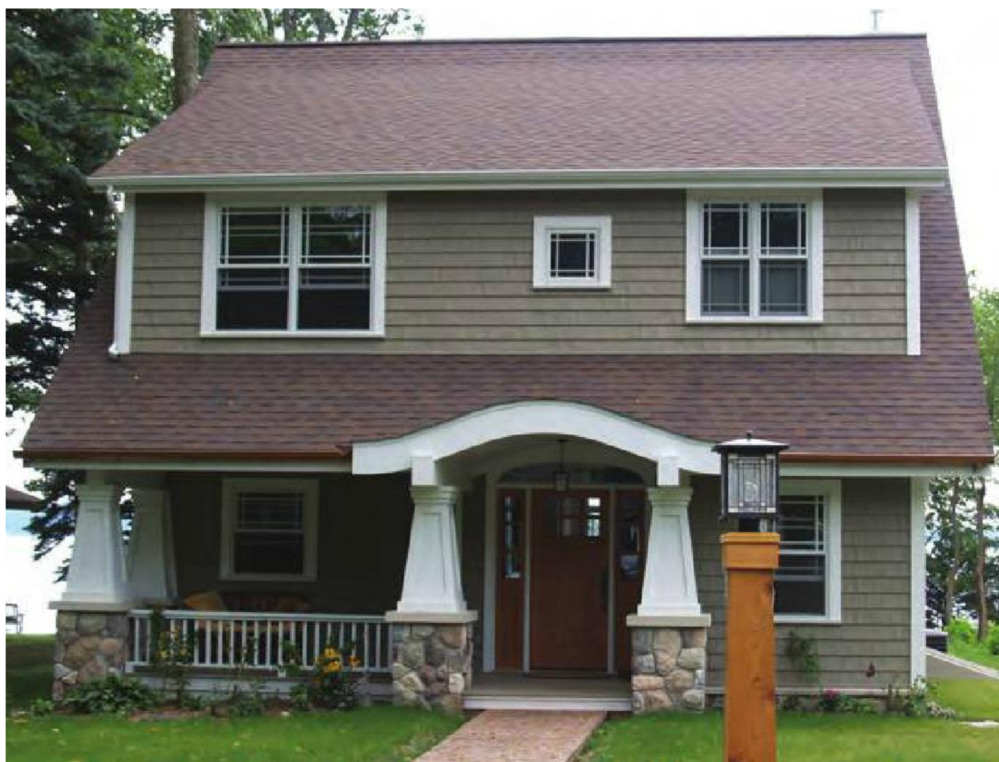
This home's Craftsman style flaunts the skill of the carpenter, who used traditional shake cladding on the walls and roof. Vinyl shakes were combined with dimensional composition shingles for a credible re-creation. Note the wide cellular-PVC tapered columns. The white preprimed material requires no maintenance, though you can paint it if you prefer.
