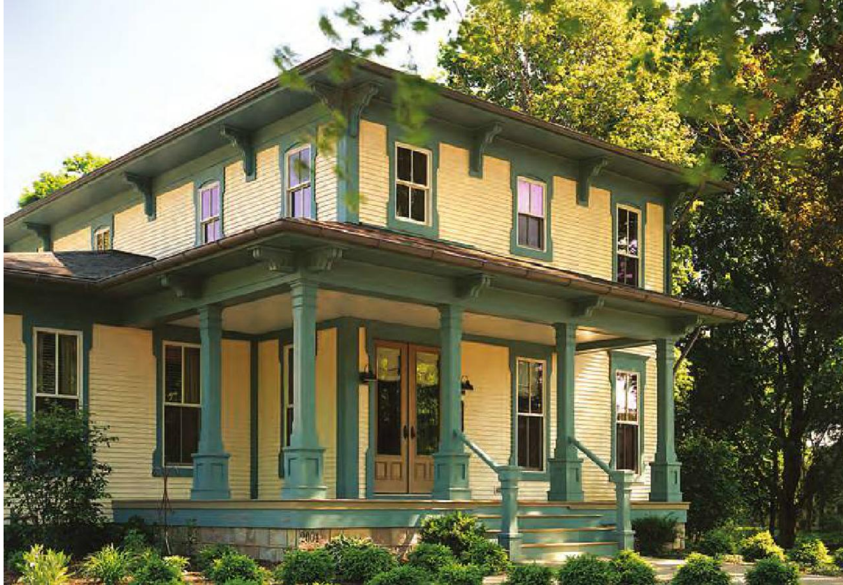
This Italianate-style home offers an example of excellent vinyl siding design and craftsmanship. The window trim and brackets are vinyl, and the columns are painted cellular PVC. Note the wide frieze board scribing the roof and the 6-in.-wide outside corners. The wide inside corners were created by vertically installing a 4-in. band board.
