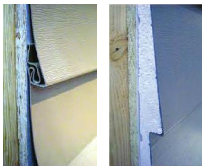
Insulated siding features a straight plank that's more attractive than the cupped appearance of traditional vinyl.
