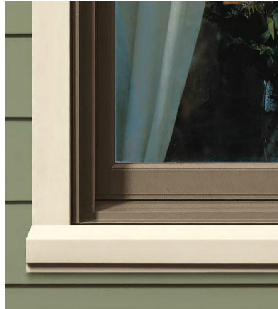
Lineals and sills are an inexpensive way to dress up vinyl siding.
