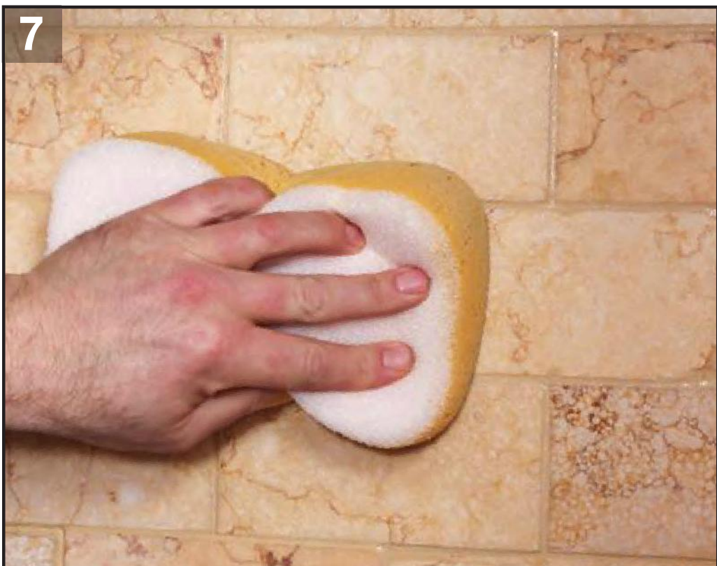
7 Let the grout sit for about 20 or 30 minutes and then wipe it off with a damp sponge. This is the time to even out any high and low spots and fill any holes you find.
