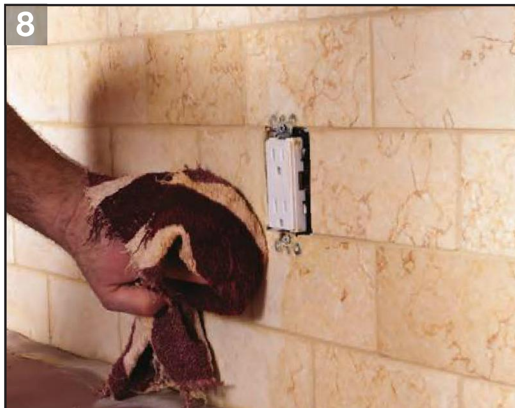
8 Let the grout sit for a half hour or so; then wipe off the haze with a damp cloth. Use a gentle touch to avoid removing grout from between the tiles.
