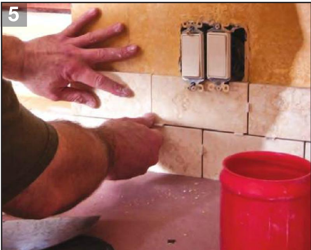
5 Use spacers between tiles. Make sure that the tongues of electrical devices sit on top of your tiles. You can cut or nip small notches for the screws if necessary.
