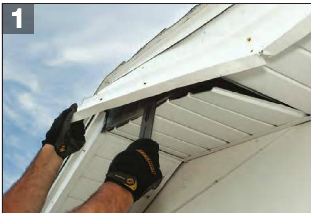
1 If your house has existing aluminum soffits, remove any damaged sections. Don't reuse old components, as they're likely to have weak spots that will tear in windy conditions.
