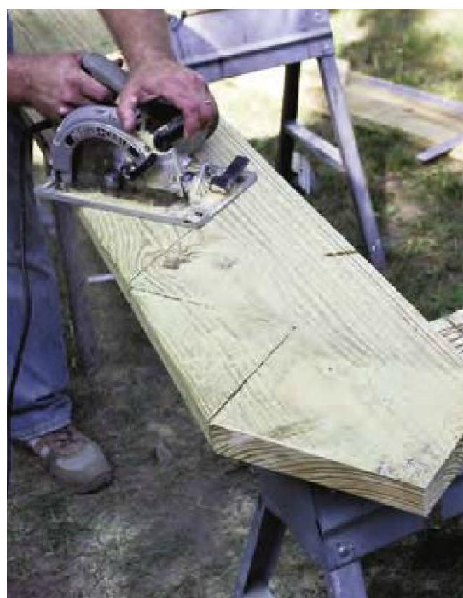
To form stair stringers, make the bulk of the cuts with a circular saw, stopping just short of the corners (left); then use a reciprocating saw to finish the cuts (right).
