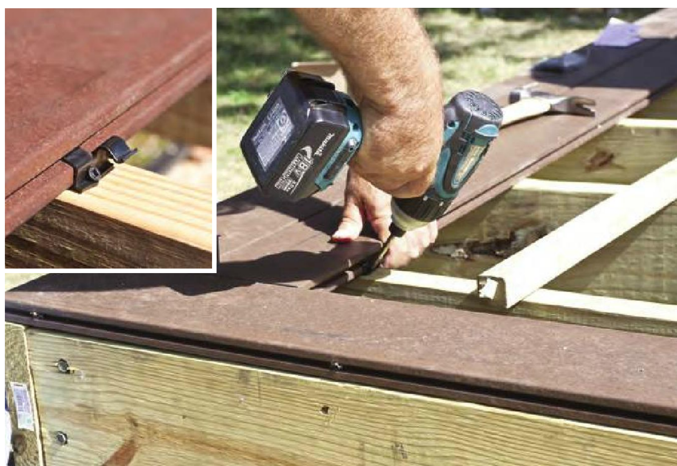
Unlike many hidden fasteners, Trex fasteners are installed from above, and they automatically set the proper gap between boards.
