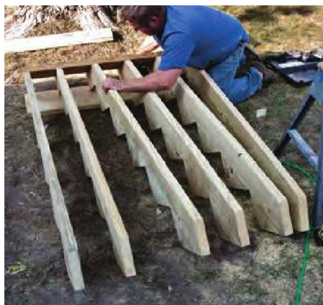
This Trex installation required six stringers spaced 9 in. OC for the stairs.
