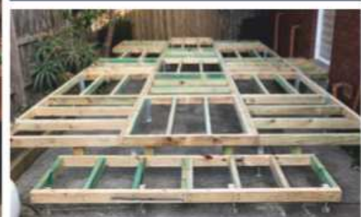
During (frames and supports)
