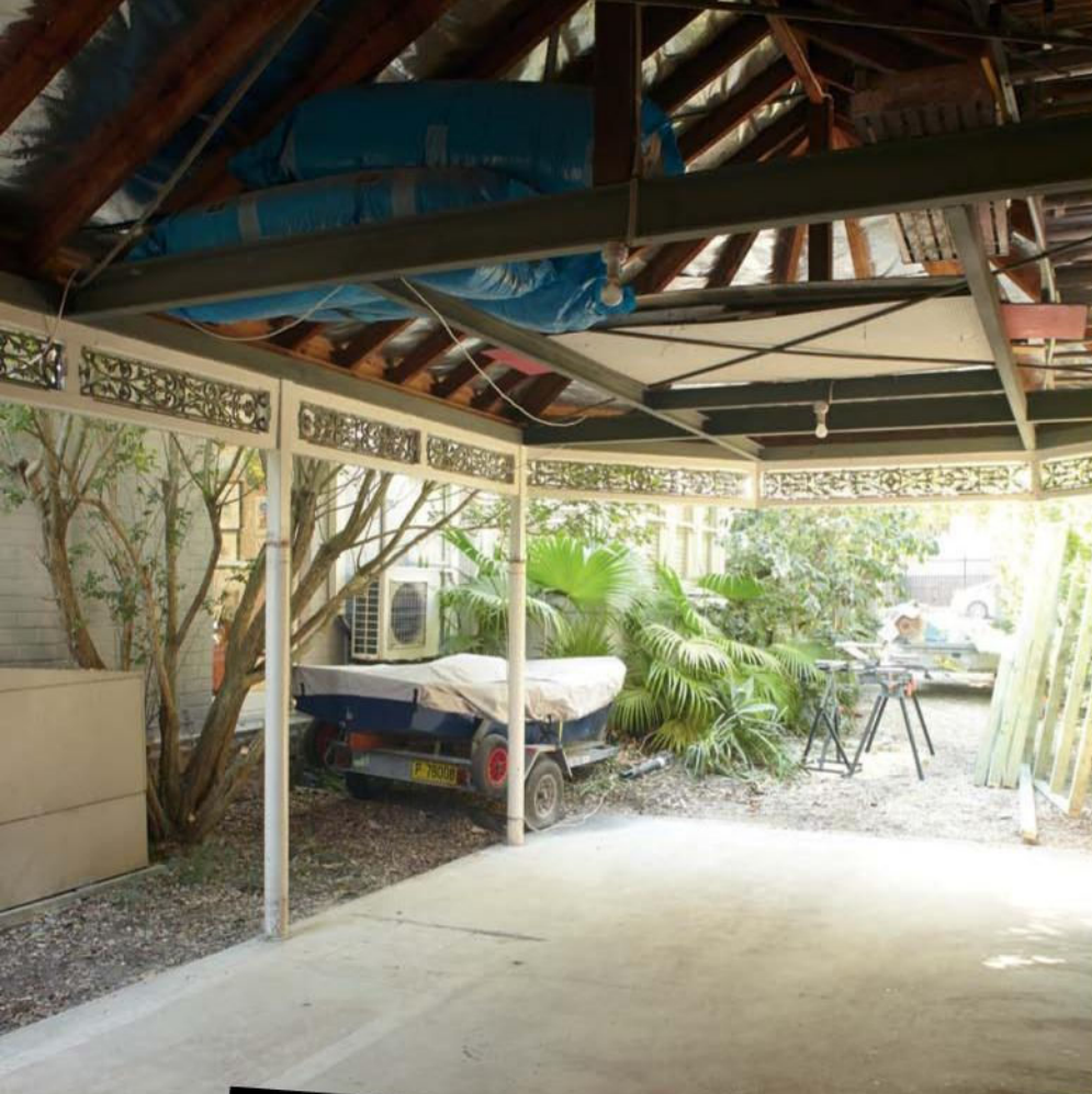
The original carport was structurally solid.
