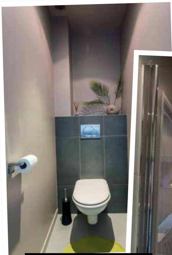
ABOVE Tiles are used to cleverly conceal the toilet cistern. RIGHT Lots of glass in the ensuite gives the illusion of spaciousness.
