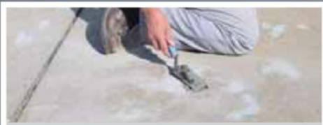
REPAIR AND PATCH
