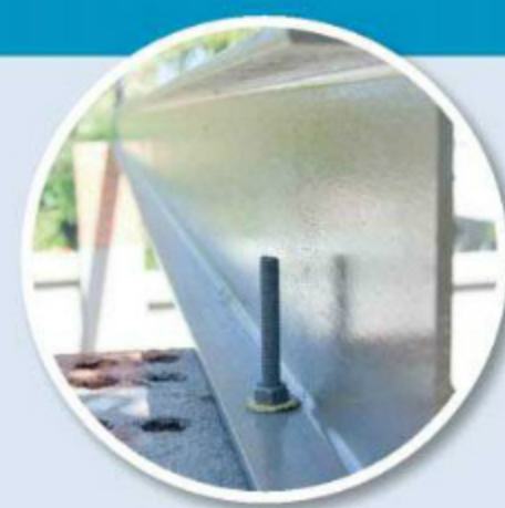
The rod was cut to length using an angle grinder and metal cutoff wheel.
