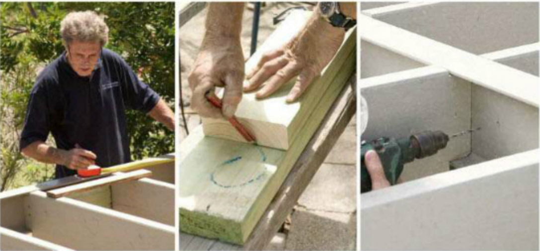
The exact spacing between the joists was measured to fit the blocking. A sliding mitresaw was used to cut the blocking to fit between the deck joists. Clearance holes 5mm in diameter were drilled through the steel web.
