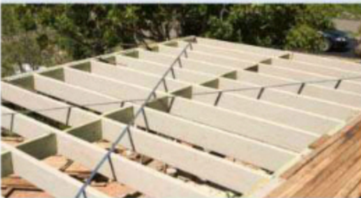
CROSS-BRACE THE DECK For further stability, metal strapping was crisscrossed corner to corner and tightened using a tensioner. This bracing was secured to the joists using 40 x 2.8mm galvanised clouts.
