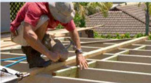
SECURE THE CENTRE BLOCKING A centre row of blocking was secured perpendicular to the joists. Every second block was offset 45mm so the blocking could be secured through the sides of the joists using nails.
