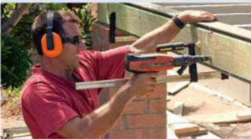
ADD THE FASCIA Treated pine was clamped to the outside of the front beam and held with Ramset nails before being secured from the reverse side with screws. Decking boards were then secured to it with nails.
