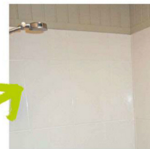
Tile paint covers the grout and provides a non-absorbent surface treatment.
