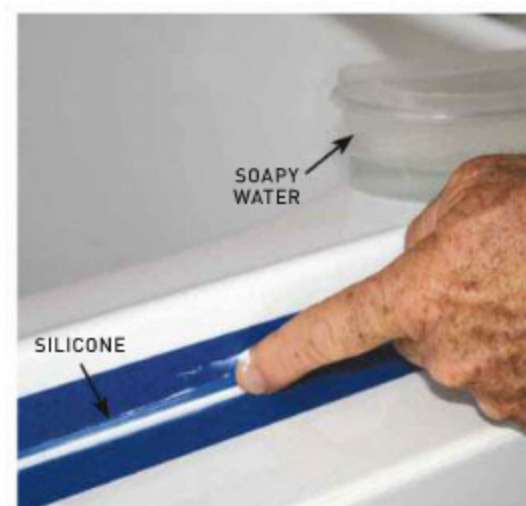
Silicone around vanities and fixtures prevents water damage and mould.
