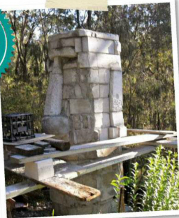
Hebel blocks on a concrete base form the main structure of the statue.
