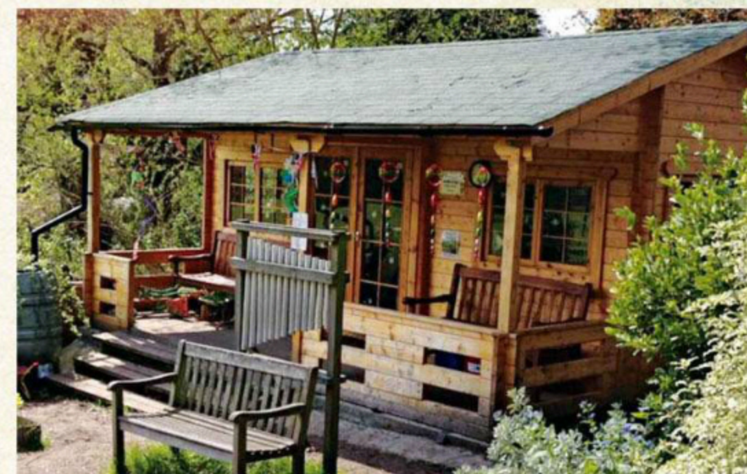
An outdoor classroom built by teachers and parents at Coombe Hill Infants School.
