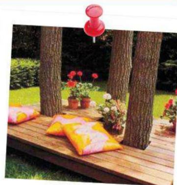
Maximise your space and build a decking platform around trees.
