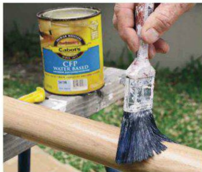
The new timber handrail was given three coats of water-based polyurethane.
