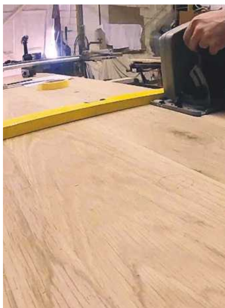
18 Pieces to make up all sides of the cabinet were marked and rough cut
