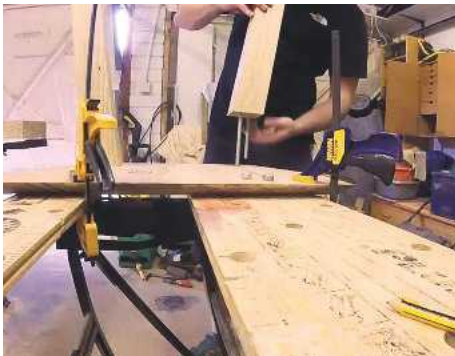
7 Threaded rod, epoxied into the legs, was then bolted to the desk top
