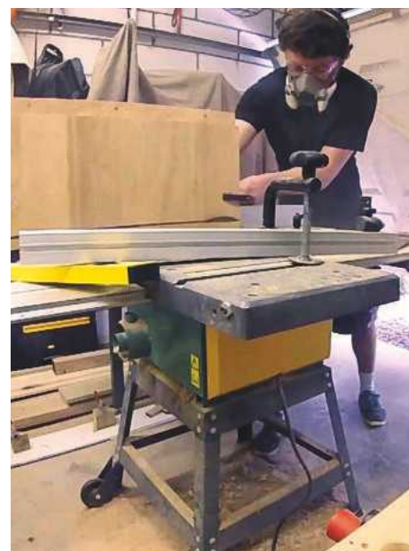
19 Mitre cuts were made on the edges of all cabinet panels
