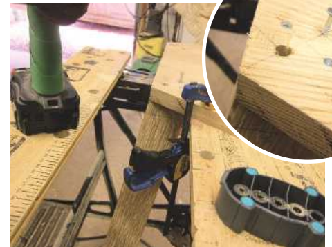
6 Screwed in place to make it easier to drill the holes for the actual mounted rods
