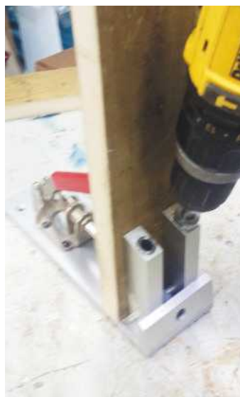
9 Drilling the pocket screws
