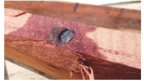
The secret of the construction: the rebar's tip
