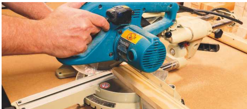
10 Using the markings from the rod, cut all the components to length
