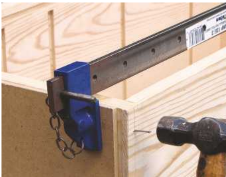
16 Pre-drill the holes to prevent splitting, and then use 20mm oval nails to assemble the joints
