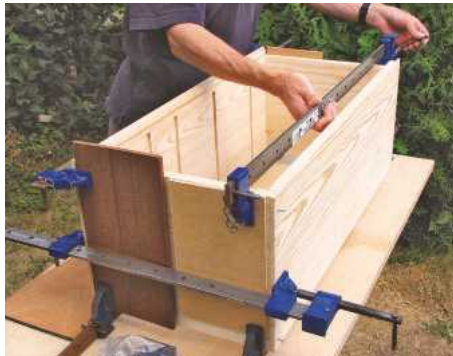
14 Do a dry run with sash clamps before gluing the carcass together. Use an exterior glue if possible
