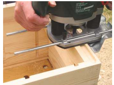
18 Rout a rebate around the inner edges for a rear panel, squaring the rounded ends with a chisel
