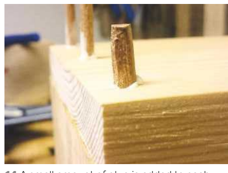
14 A small amount of glue is added to each of the holes with the dowel put a little way in
