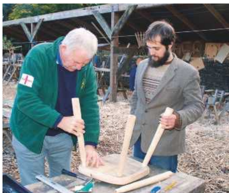
Adjusting leg tenons so they fit tightly into the seat mortises, assisted by tutor Pete Murray
