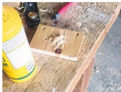
17 I mixed up some sawdust with glue and rubbed it into the gaps
