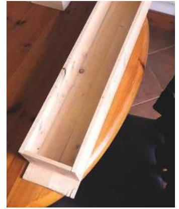
25 Well attached but the base is protruding
