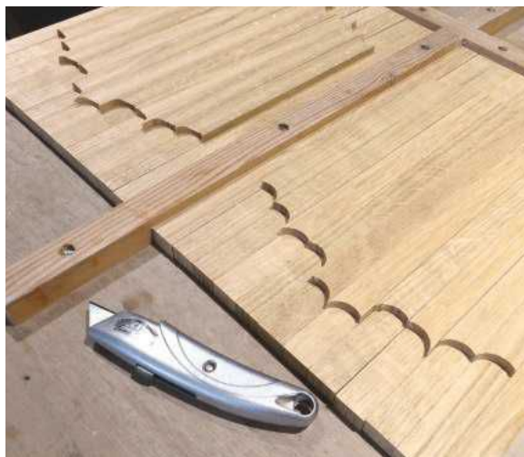
3 The ends cut. Some feathery ends need to be knifed or chiselled back
