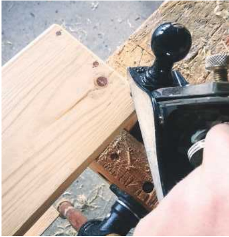
18 Using a plane to chamfer the edges
