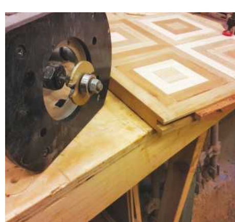
12 Cut spline joints and add a bevel using a router
