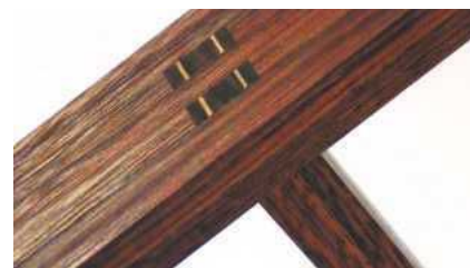
A pair of through wedged tenons
