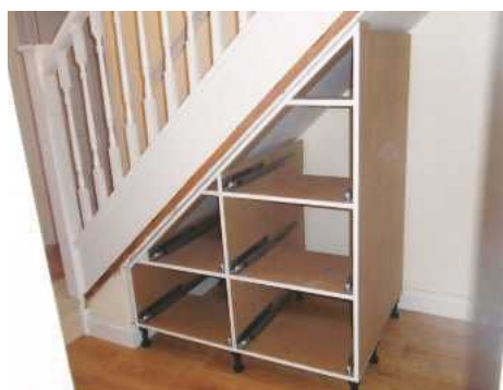
16 The frame in situ with the plinth leg
