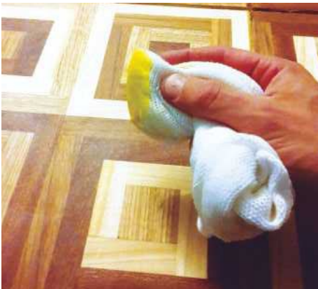
19 Apply wax according to the instructions
