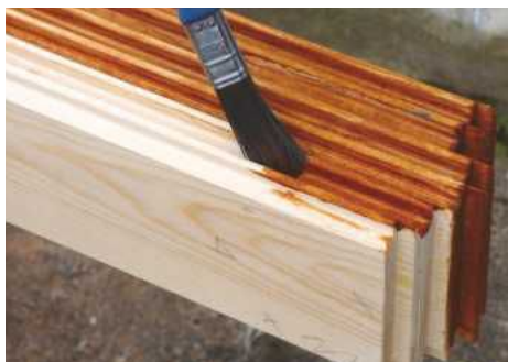
22 Before nailing the boards to the gate, paint all tongues and grooves with a couple of coats of your chosen finish
