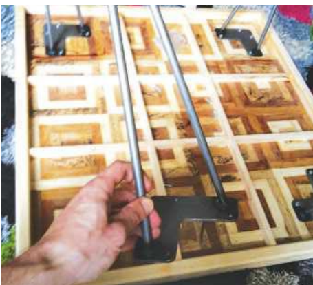
20 Hairpin legs screw into the underside
