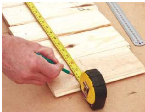
19 Fit offcuts together loosely and measure their overall width. Both outer boards will probably need to be ripped to size
