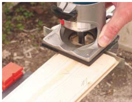
21 The underside of the top rail is also grooved to accept the matchboard. Rout rebates along the top edge of each board
