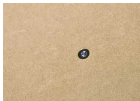
8 Conformat screw in place
