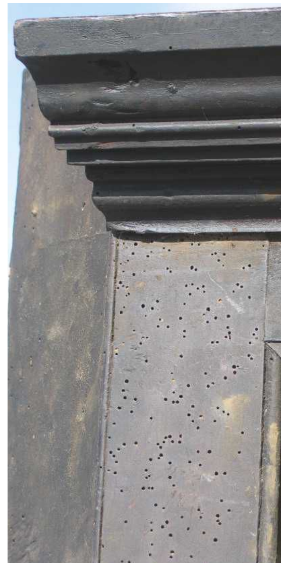
Extensive woodworm damage
