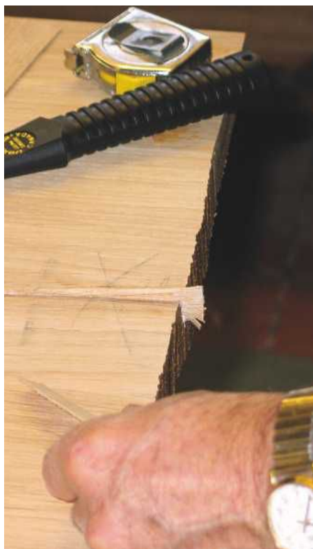
Filling splits with solid wood
