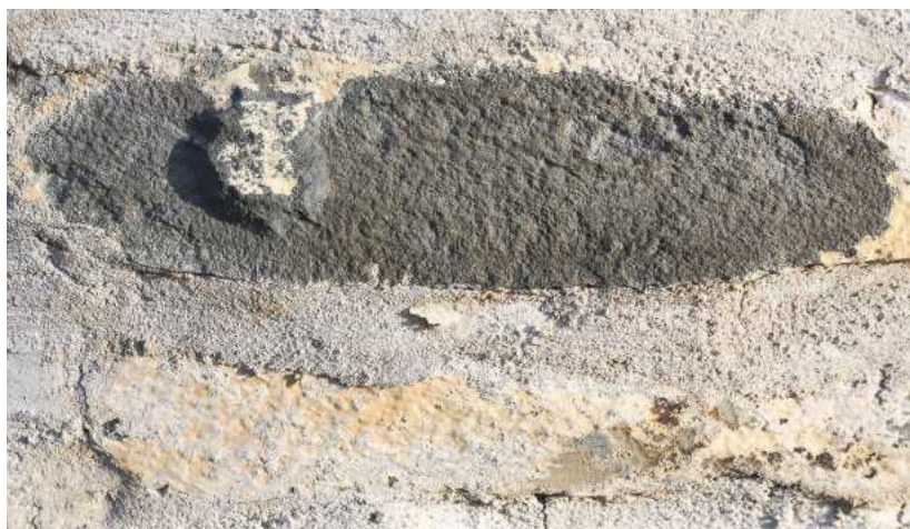
PIC 1. Drastic action: the sodium hydroxide gel lifted off even the heaviest of the masonry paint (the yellow paint on the stone at the bottom of the picture), tho' it wasn't pleasant to use
