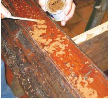
Filling woodworm holes – a thankless task!
