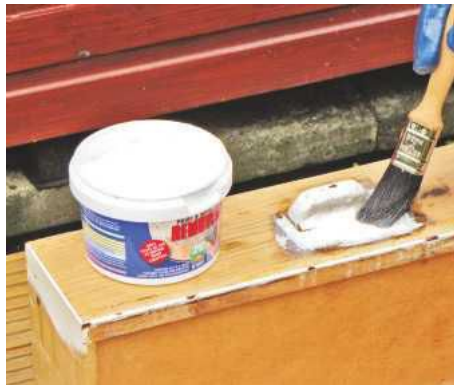
You'll need at least two applications of chemical stripper
