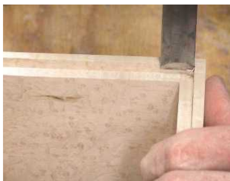
PIC 23. Cleaning up the ends of the rebate using a chisel
