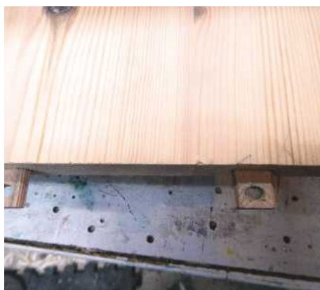
PIC 6. Dowel holes enlarged for movement
