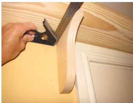
STEP 19. Slide each bracket down over its screws. Lift the shelf into place, check for square and proceed to mark the housings
