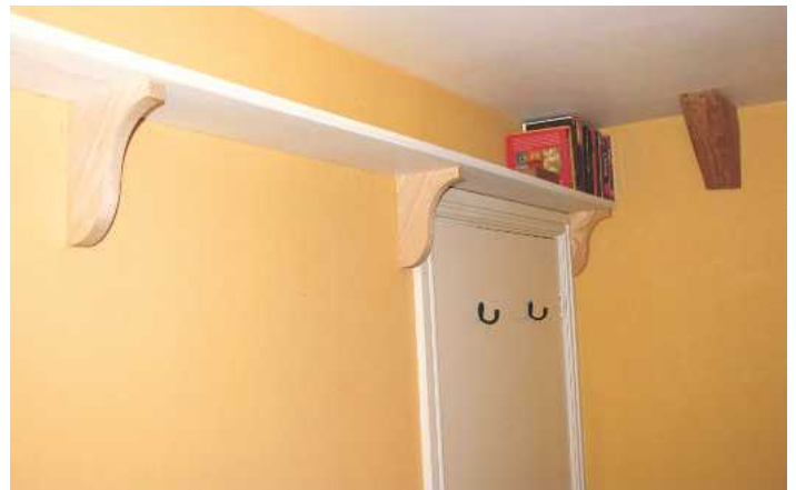
The height of the shelf is dictated by the door opening and it had to sit atop of the architrave
