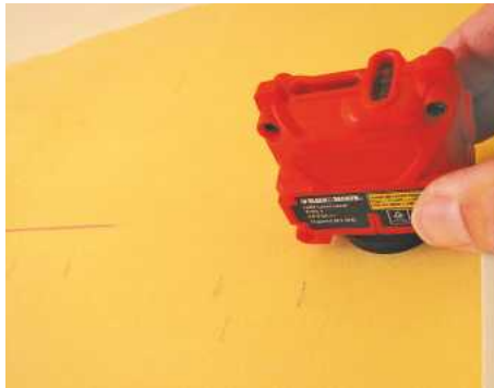
STEP 2. Use a laser level to continue the shelf height along the length of the wall
