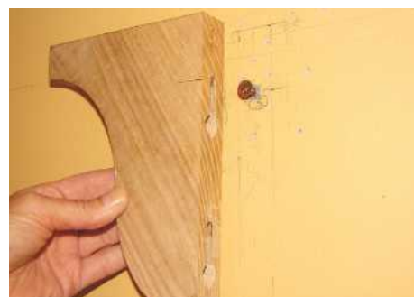
STEP 18. Carefully mark bracket positions on the wall and insert 5mm screws, checking each slot length
