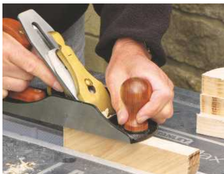
STEP 13. You'll probably need to trim the straight edges of each bracket with a bench plane
