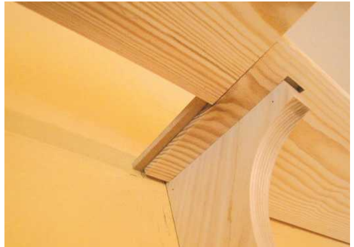
The height of the shelf is dictated by the door opening and it had to sit atop of the architrave
