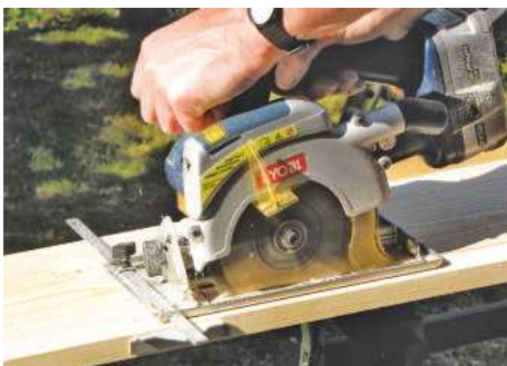
STEP 4. Cut the timber down to width if necessary with a circular saw. Clean up the edges with a bench plane
