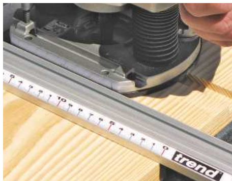
STEP 20. Rout a stopped housing on the underside of the shelf for each bracket. Use a guide fence to ensure accuracy
