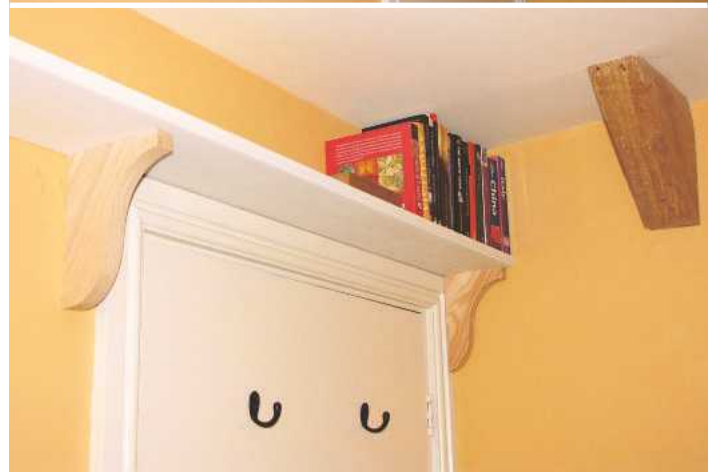
With an overall length of 3.5m it made sense to use two pieces of timber, as the shelf's rear edge had to be scribed to fit the rather undulating wall
