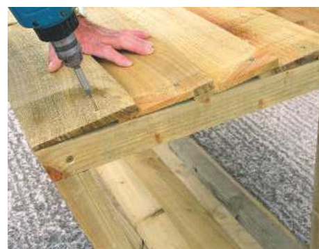
Fixing feather-edged boards
