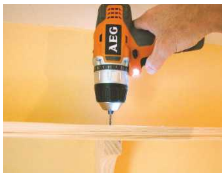
STEP 23. Insert the loose tongue and slide the shelves into place. Drill a single screw hole into each bracket
