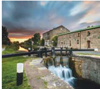
PIC 6. Every year, about 100 of the canal system's 1,580 oak lock gates are replaced
