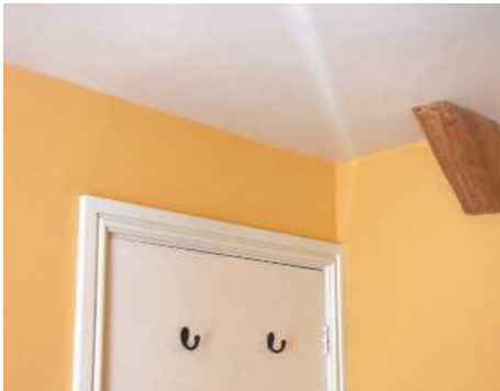
STEP 1. As the shelf was to sit across the architrave there were no decisions to make regarding final height
